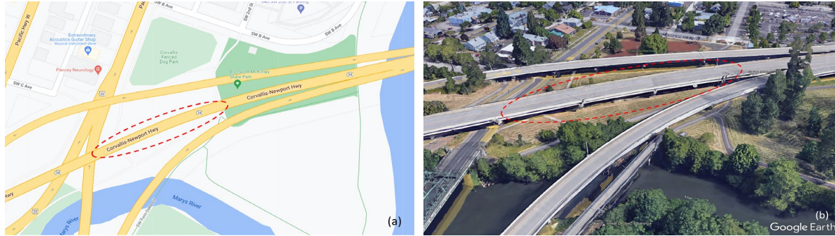
Figure 4.1. The location of the case study site in Corvallis, Oregon. (a) The bridge location on Google Maps; (b) 3D scene of the bridge on Google Earth.
