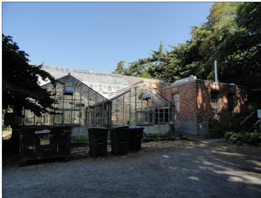
Figure 7-11. Plant Lab, view northeast.
