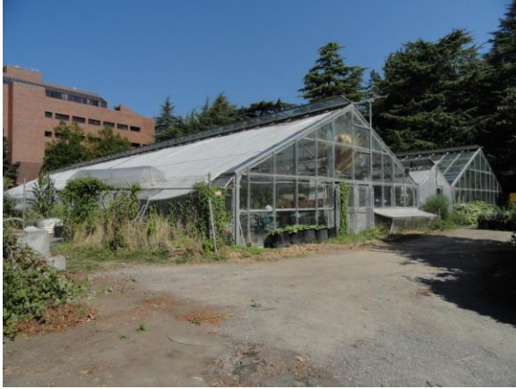
Southeast elevation, view to the north 2014
