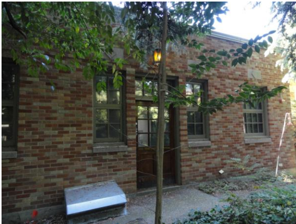
Primary facade of brick offices, view to the southwest 2014
