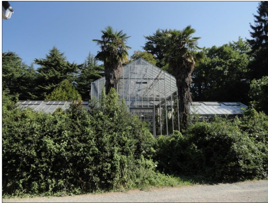
Figure 7-10. Plant Lab, view north.
