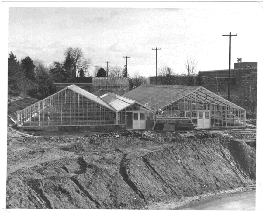
Figure 8-2. Historic photo of the Botany Greenhouse under construction, 1947 (UW Special Collections).
