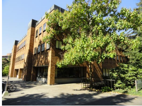
Southeast corner, view to the west 2014
