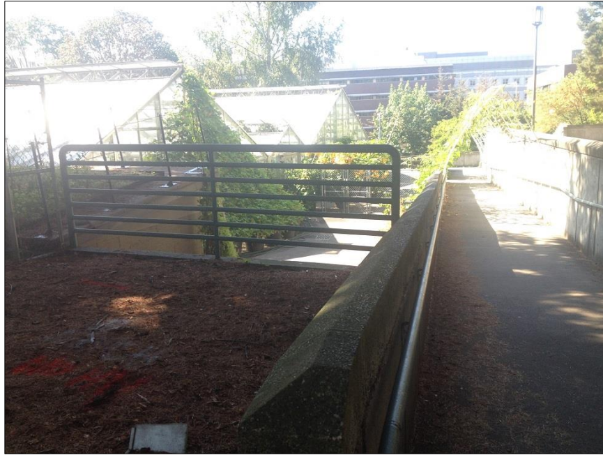
Figure 7-2. View of west end of Greenhouses from near Stevens Way (view southeast).
