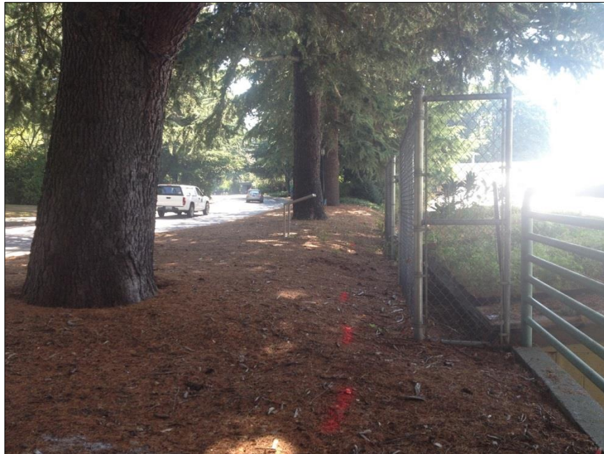
Figure 7-3. Electric utility marked south of W Stevens Way NE, view east from SP5 location.
