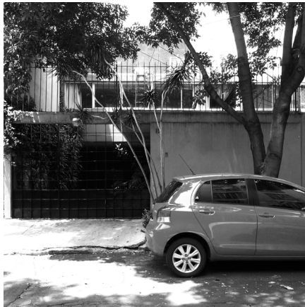
a The existing house is a concrete frame structure built in the late 1950s
