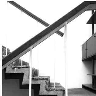
D A double-height open stair connects both floors.
