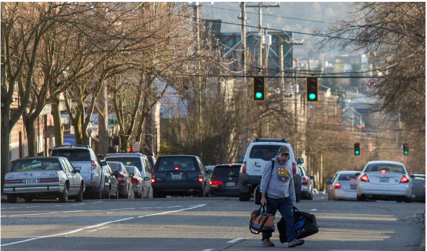
Fig. 4-23: Roosevelt Way NE, facing south from NE 75th St. The lack of functional crosswalks along the corridor force people to cross at unsignaled, mid-block locations, posing a safety concern for pedestrian, bicyclists, cars, and buses.
