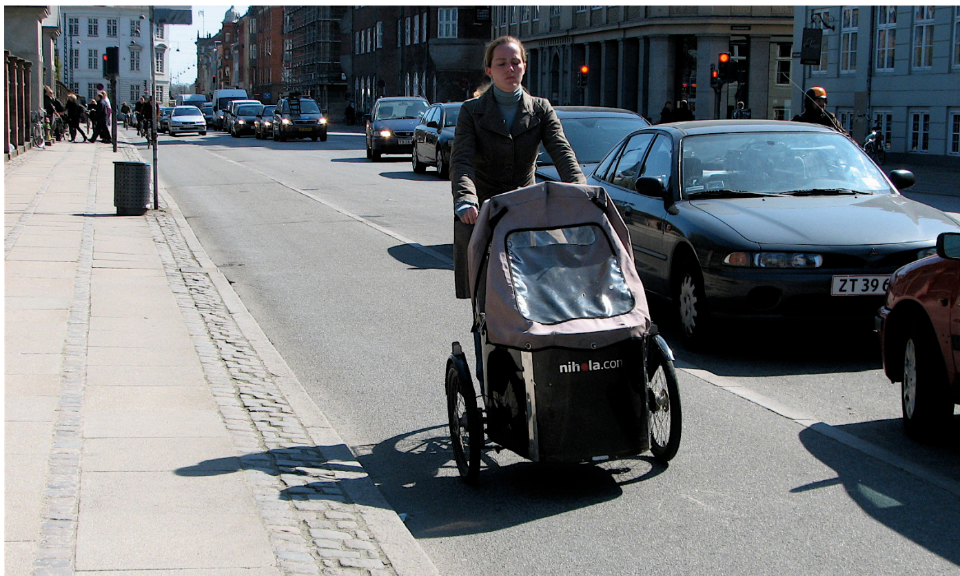
Fig. 5-15: An example of a raised, protected bike lane in Copenhagen, Denmark. Photo from Wikipedia
