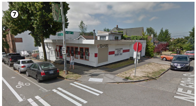
Fig. 4-9: 6718 Roosevelt Way NE. Image from Google Street View.
