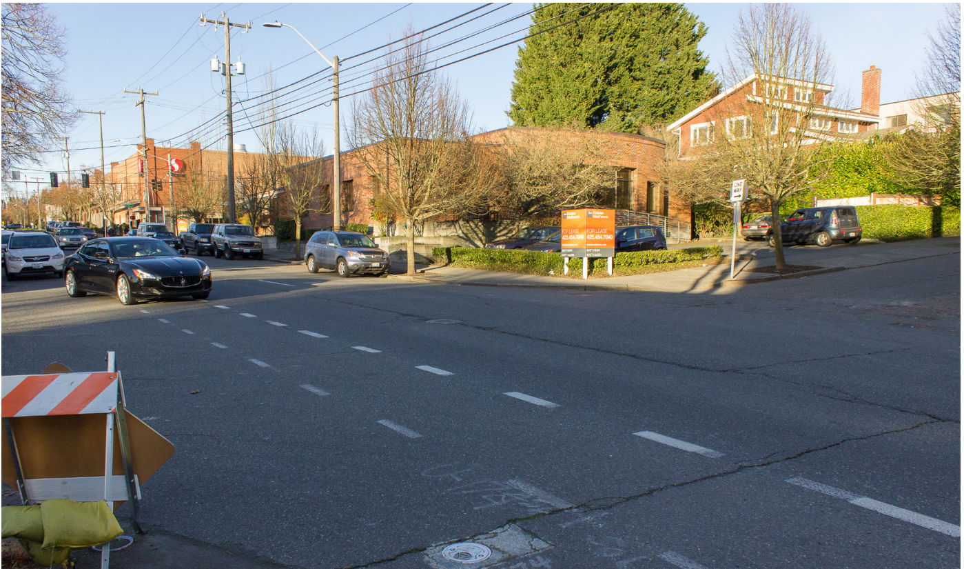
Fig. 4-22: Roosevelt Way NE, facing northeast from NE 72nd St. In addition to subpar sidewalks, the corridor is lacking in appropriate across-the-street pedestrian safety. This intersection at NE 72nd St has no painted crosswalks, giving no visual indication to cars that it is, in fact, legal for pedestrians to cross here.
