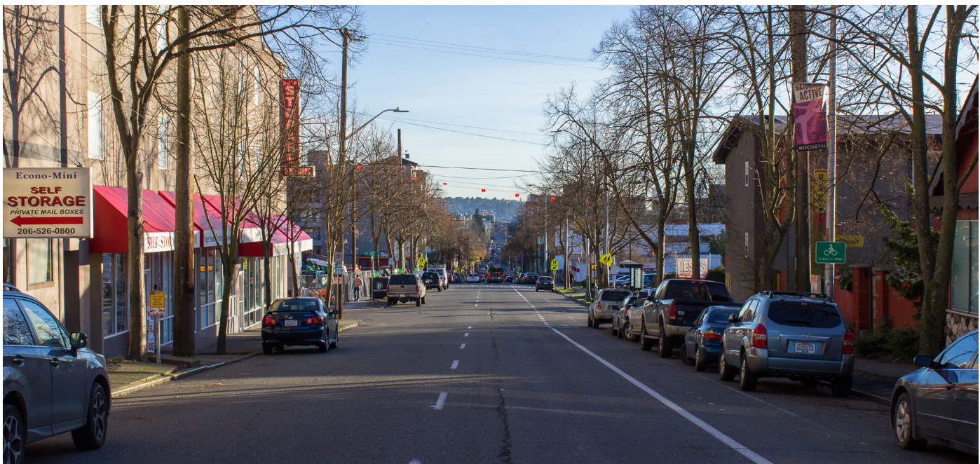
Fig. 4-19: Roosevelt Way NE, facing south from NE 69th St. The typical channelization along the corridors (from left to right: a parking lane, two travel lanes, a bike lane, and a parking lane) can be seen continuing almost uninterrupted all the way to the University bridge, about 30 blocks south.
