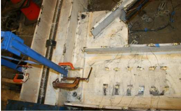
Figure 5.141 NCBF1-R4 Undamaged North Connection
