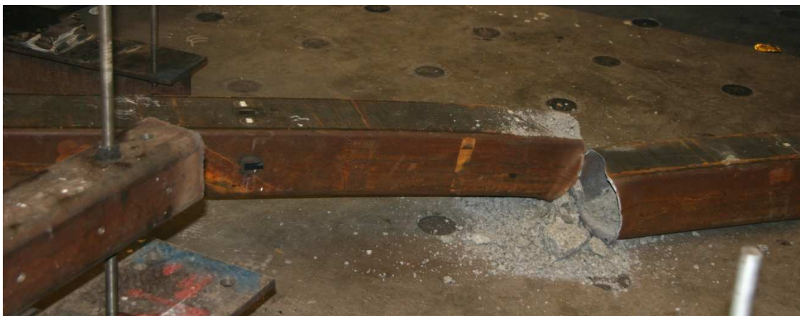
Figure 5.235 Brace Fracture - BF
