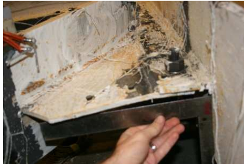
Figure 5.112 North Gusset Plate Downward Bending at Shear Tab
