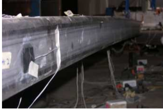
Figure 5.59 Initial Brace Buckling - B1
