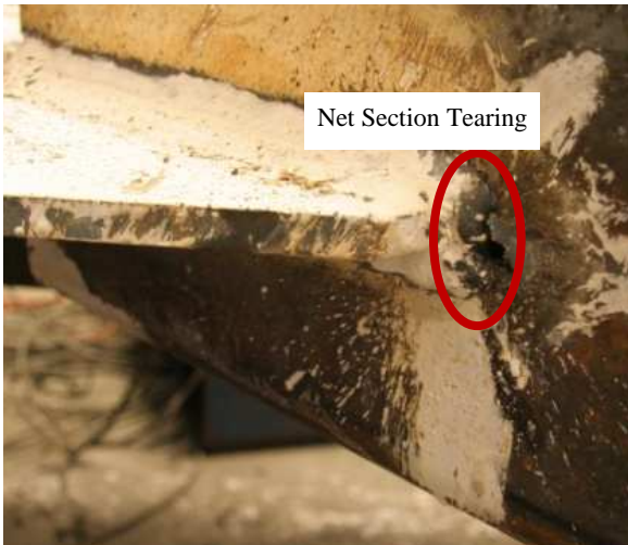
Figure 5.195 BNS at SW Gusset, South Wall
