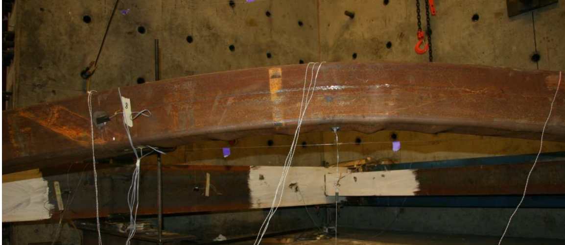
Figure 5.203 Bulges in Brace Bottom Flange
