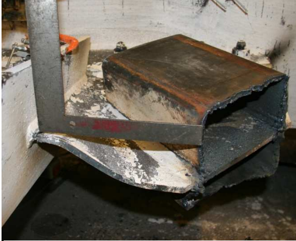
Figure 5.238 Buckling of South Gusset Plate
