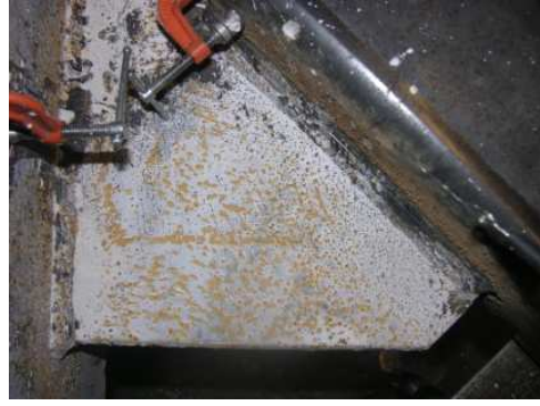
Figure 5.69 South Gusset Plate - Y2
