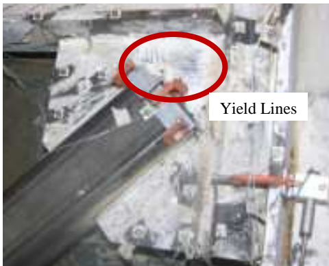
Figure 5.60 North Gusset Plate - Y1
