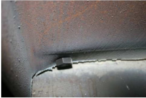
Figure 5.120 Upward Bending of N Beam Web
