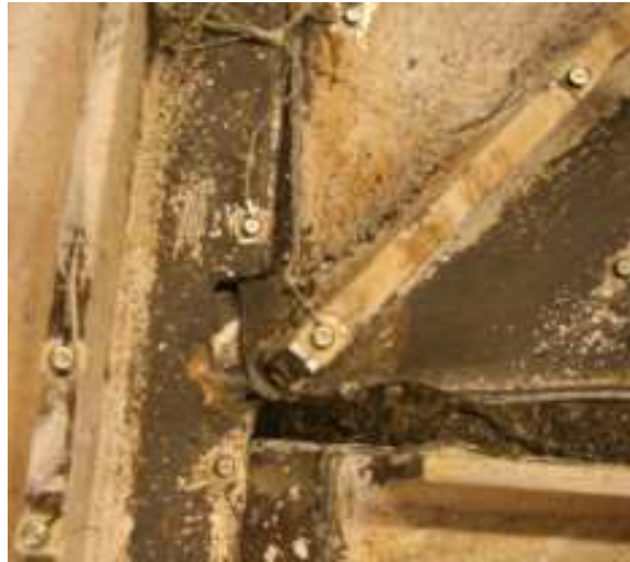
Figure 5.137 North shear tab - MT
