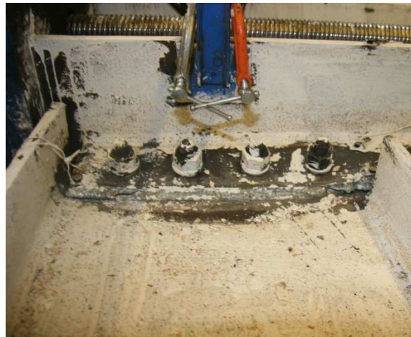
Figure 5.241 W3 in North Beam-to-Shear Tab Weld
