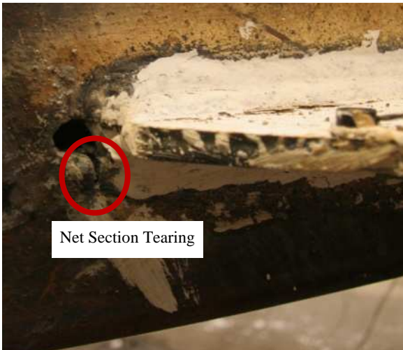
Figure 5.194 BNS at NE Gusset, South Wall
