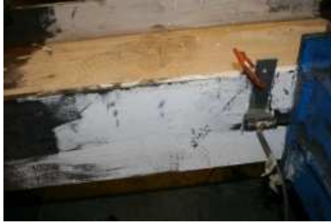
Figure 5.108 North Flange, North Beam - Y1
