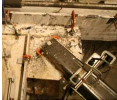
Figure 5.88 South Gusset Plate - Y3
