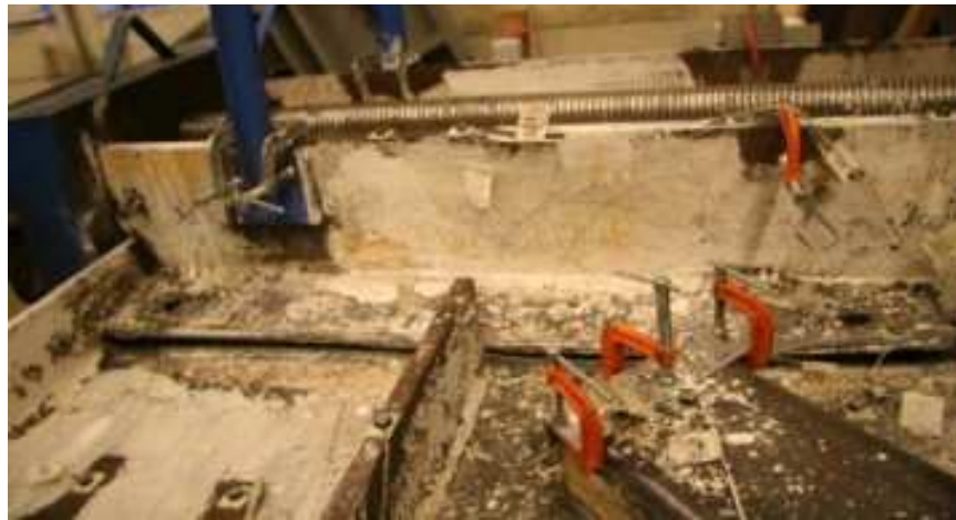
Figure 5.84 Complete Fracture of the North Shear Tab Weld
