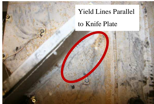
Figure 5.146 Y1- Initial Yielding in North Gusset Plate
