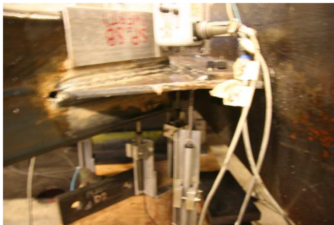
Figure 5.42 Downward Bending of South Gusset Plate
