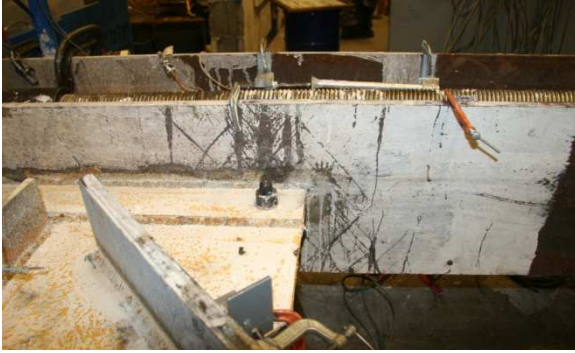
Figure 5.143 Existing Damage to West Column Flange
