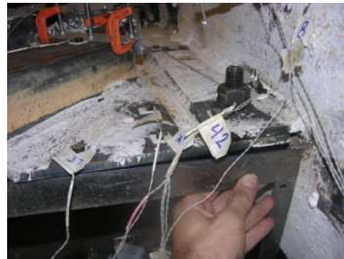
Figure 5.66 North Gusset Plate Downward Bending
