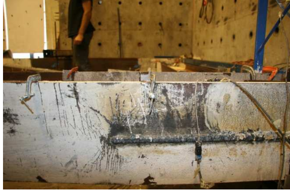
Figure 5.155 West Column, West Flange - Y1
