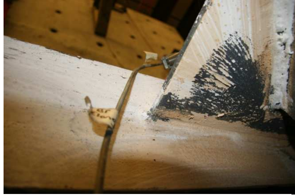
Figure 5.209 South Gusset-to-Beam Weld - W1
