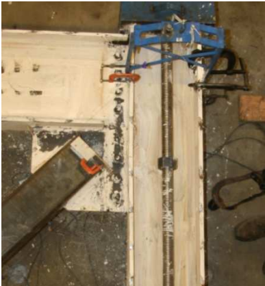
Figure 5.3 Gusset Plate Y3 NCBF1-R5
