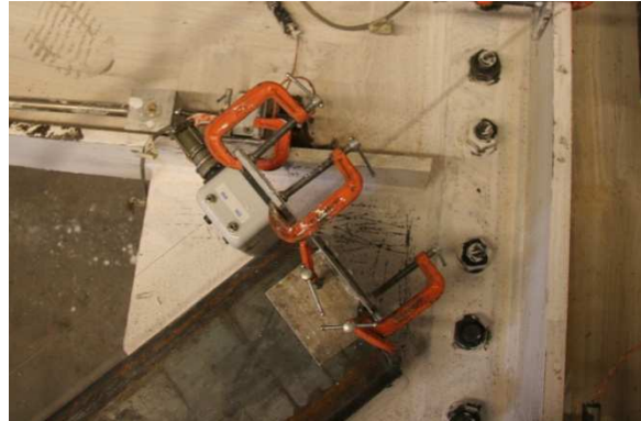
Figure 5.183 Yielding in South Gusset - Y2
