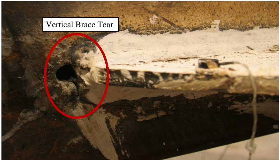
Figure 5.14 Brace Net Section Tearing - BNS NCBF1-R5
