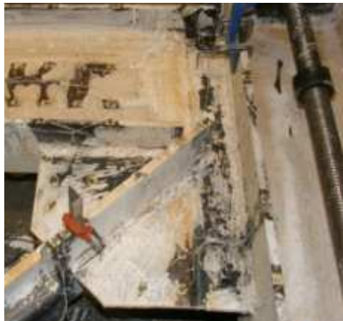
Figure 5.107 North Gusset Plate and Shear Tab - Y3
