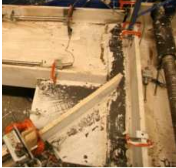
Figure 5.139 Final Damage to South Connection
