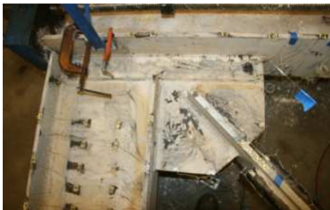
Figure 5.158 North Gusset Plate - Y2
