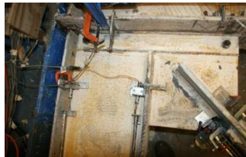
Figure 5.159 South Gusset Plate - Y2
