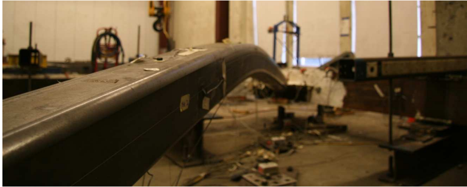
Figure 5.11 Severe Brace Global Buckling - B3 NCBF1-R2
