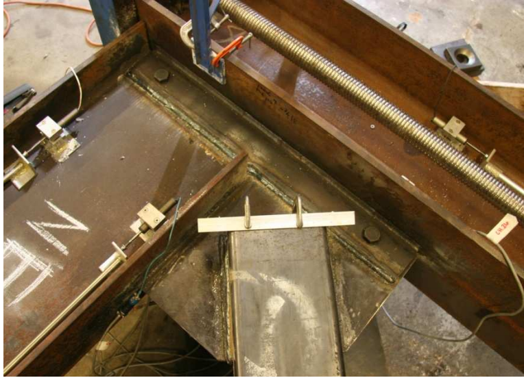
Figure 5.32 NCBF Undamaged North Connection
