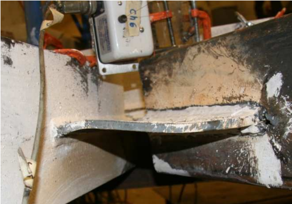
Figure 5.226 Bending of South Gusset - East
