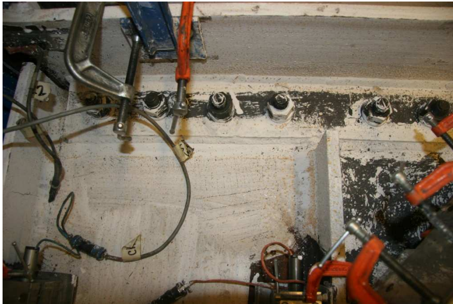
Figure 5.210 North Beam Web at South Connection - Y1
