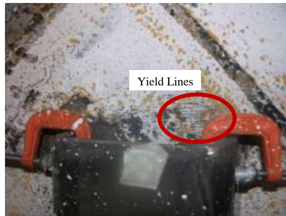
Figure 5.64 South Gusset Plate - Y1
