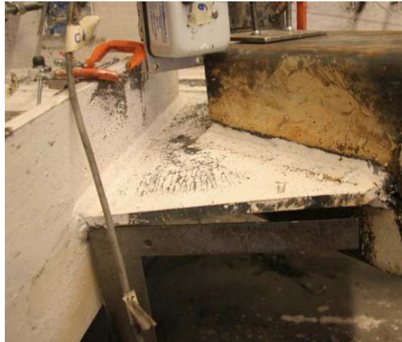
Figure 5.200 Bending of South Gusset Plate
