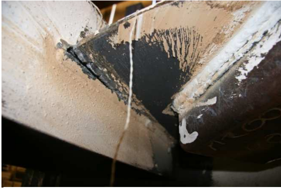
Figure 5.208 North Gusset-to-Beam Weld - W3
