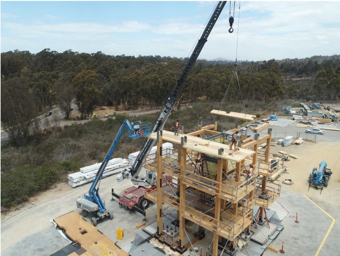
Figure 3.8: Crane Lifting Panel
