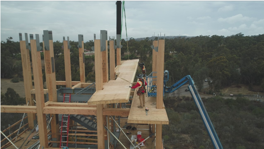
Figure 3.9: Workers Guiding Panel Into Place
