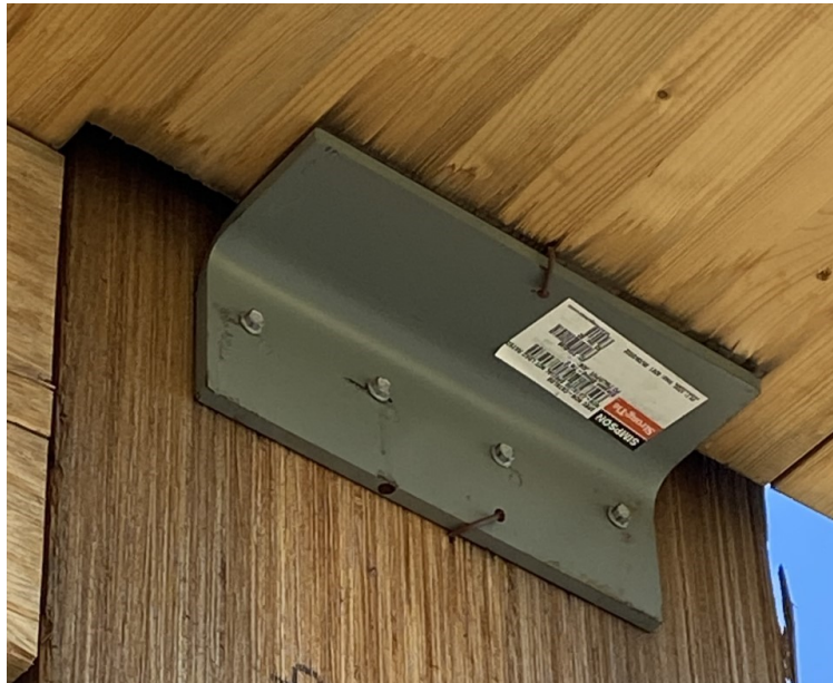
Figure 3.3: Weak Axis Support Angle
