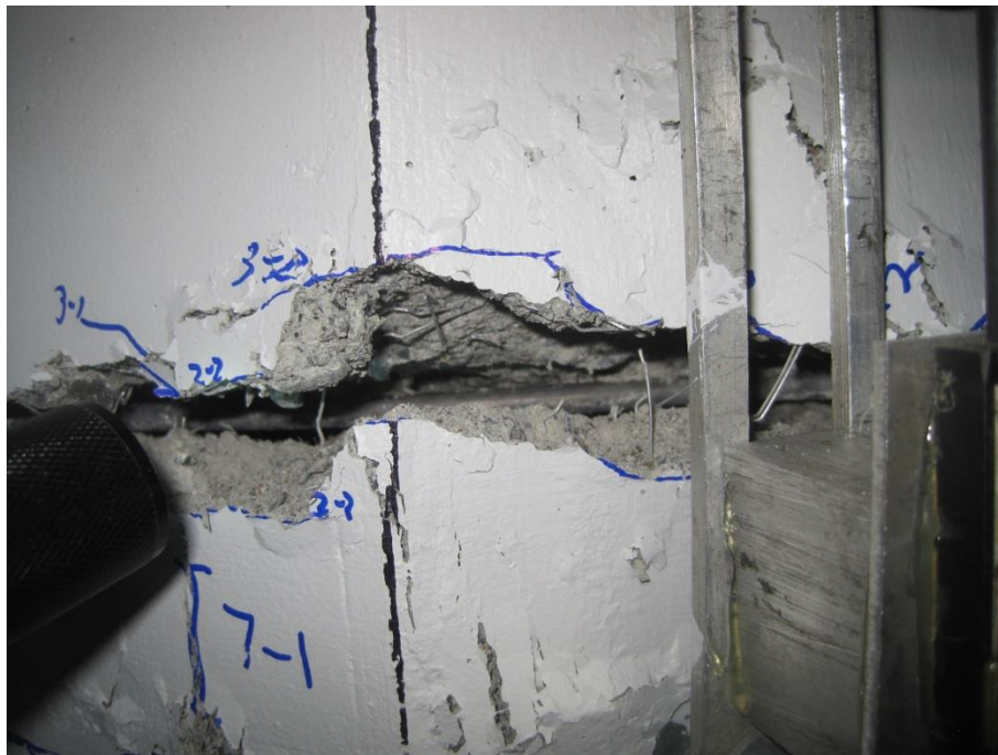
Figure C - 11: Large crack in concrete core, cycle 8-2.
