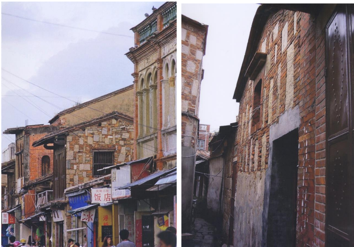
Fig. 32: Photos about some property's gable walls in West Street area (Werkhart International, 2005).
