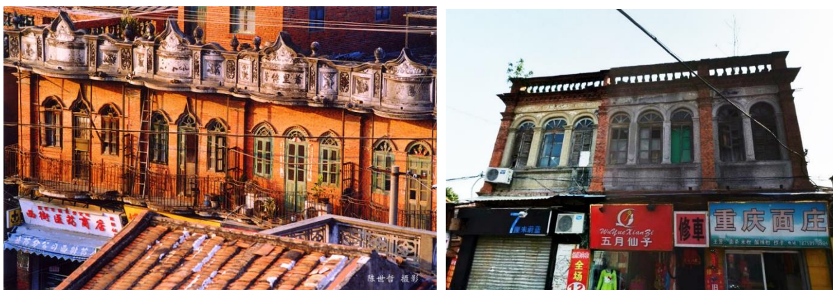
Fig. 6: Yang lou properties on West Street (Source: the Quanzhou exhibition march 1999; Major producer: Johan Nilsson, Tan Ying, & Daniel B. Abramson).
