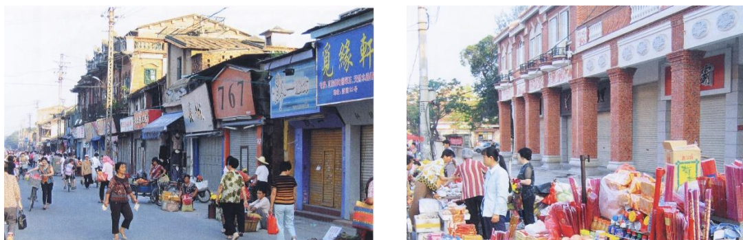
Fig. 2: Comparing the original street view (picture on the left) with the street-widening part on West Street (picture on the right) (Idziorek, 2008, p. 53). The Street widening projects demolished and rebuilt the properties along the street, which diminished the diversity and activities emerging from individual actions.
