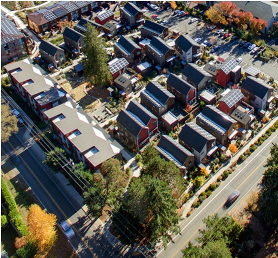
Figure 3.3. Photo of Green Built Community Solar Arrays.
