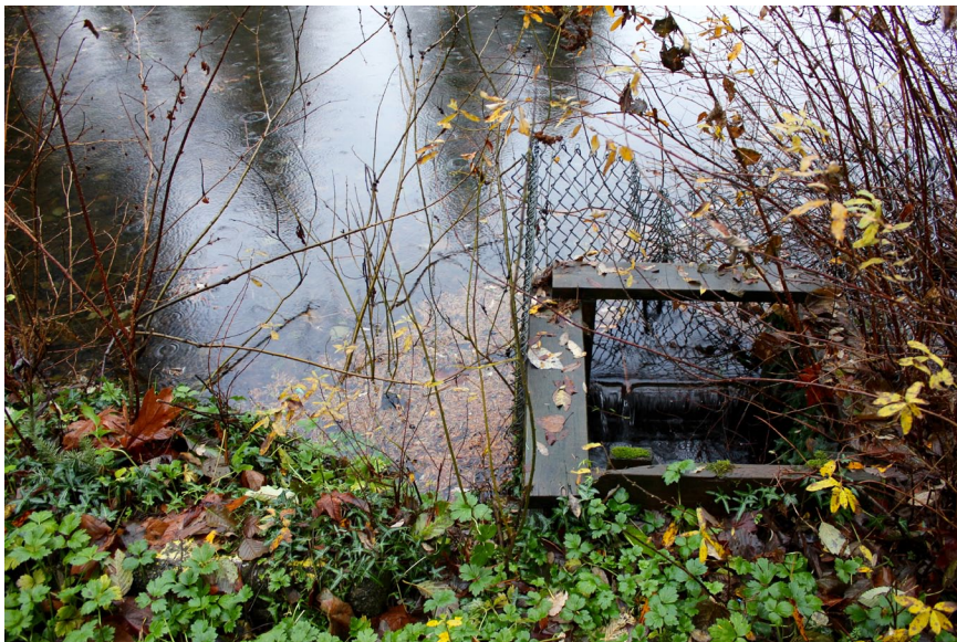
The small man-made dam that regulates the height of the lake and represents the one outflow point of the lake. Stream 0006 emerges from this dam.
