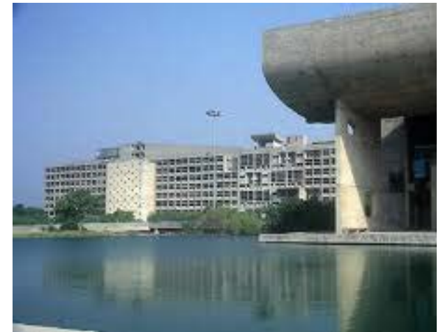
Figure 3.8 -Capitol Complex, The Secretariat Building,Chandigarh
