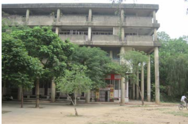
Figure 4.32- site conditions, Adjoining Buildings
