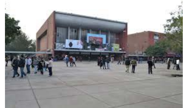
Figure 3.28- Neelam Theatre, Sector 17, Chandigarh
