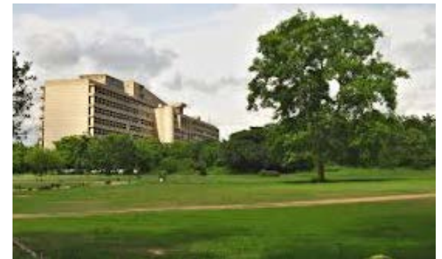
Figure 3.9 - Capitol Complex, The Secretariat Building,Chandigarh
