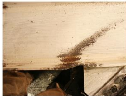
a) Extensive Local Beam Yielding of BRB05
