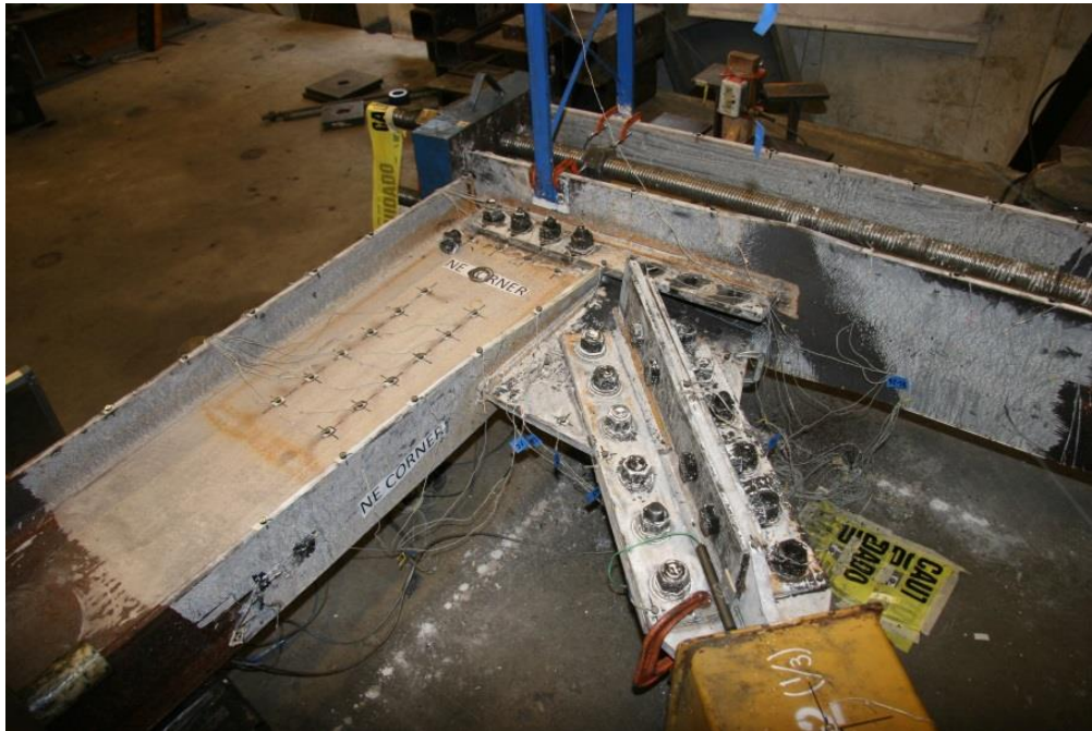
Figure 5-92: Bolt Fracture of NE Gusset Plate-to-Shear Plate Bolts (5.2%)
