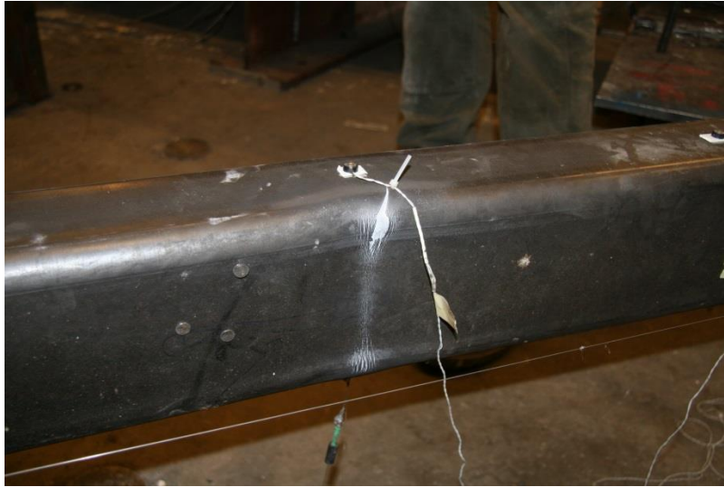
Figure 5-40: Brace Tearing (PS B4-BT, 3.9%)
