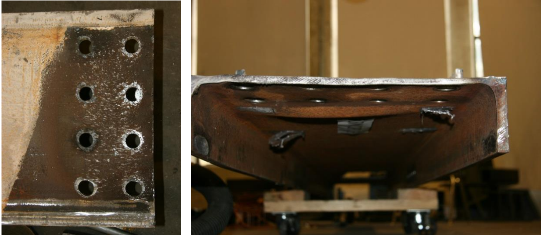
Figure 5-80: Damage to the SW Beam Web at End of Test
