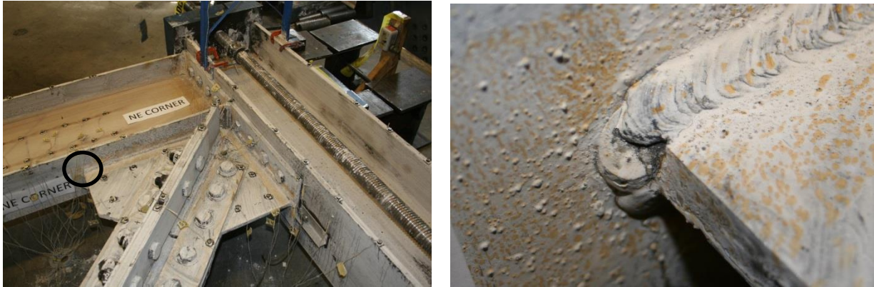
Figure 5-49: Initial Weld Cracking in the NE Beam-to-Gusset Plate Weld (PS W1, 2.5%)
