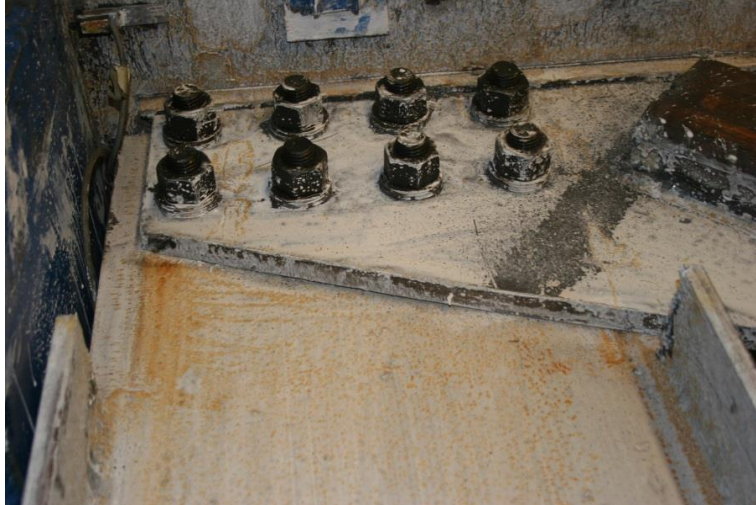
Figure 5-71: Local Web Buckling in SW Corner (PS LB1, 3.7%)
