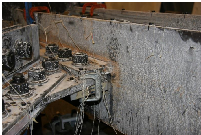
Figure 5-85: Initial Yielding in the E Column (PS Y1-PH, 1.0%)
