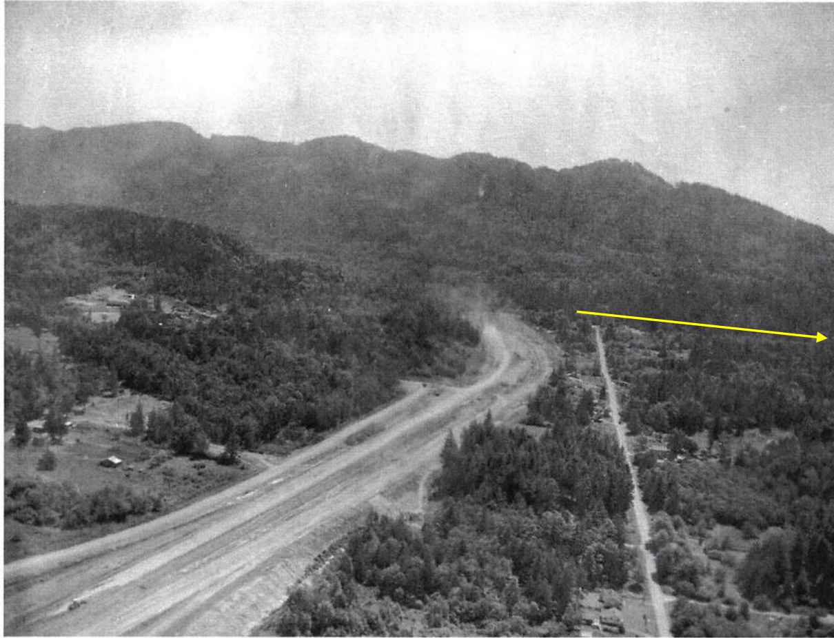
Figure 8: Southeast-facing photograph showing loose sediment production during the Interstate 5 construction. Chuckanut Creek location and drainage direction are indicated by the yellow arrow. Image taken by Jack Carver around 1963 and provided courtesy of the Whatcom Museum.
