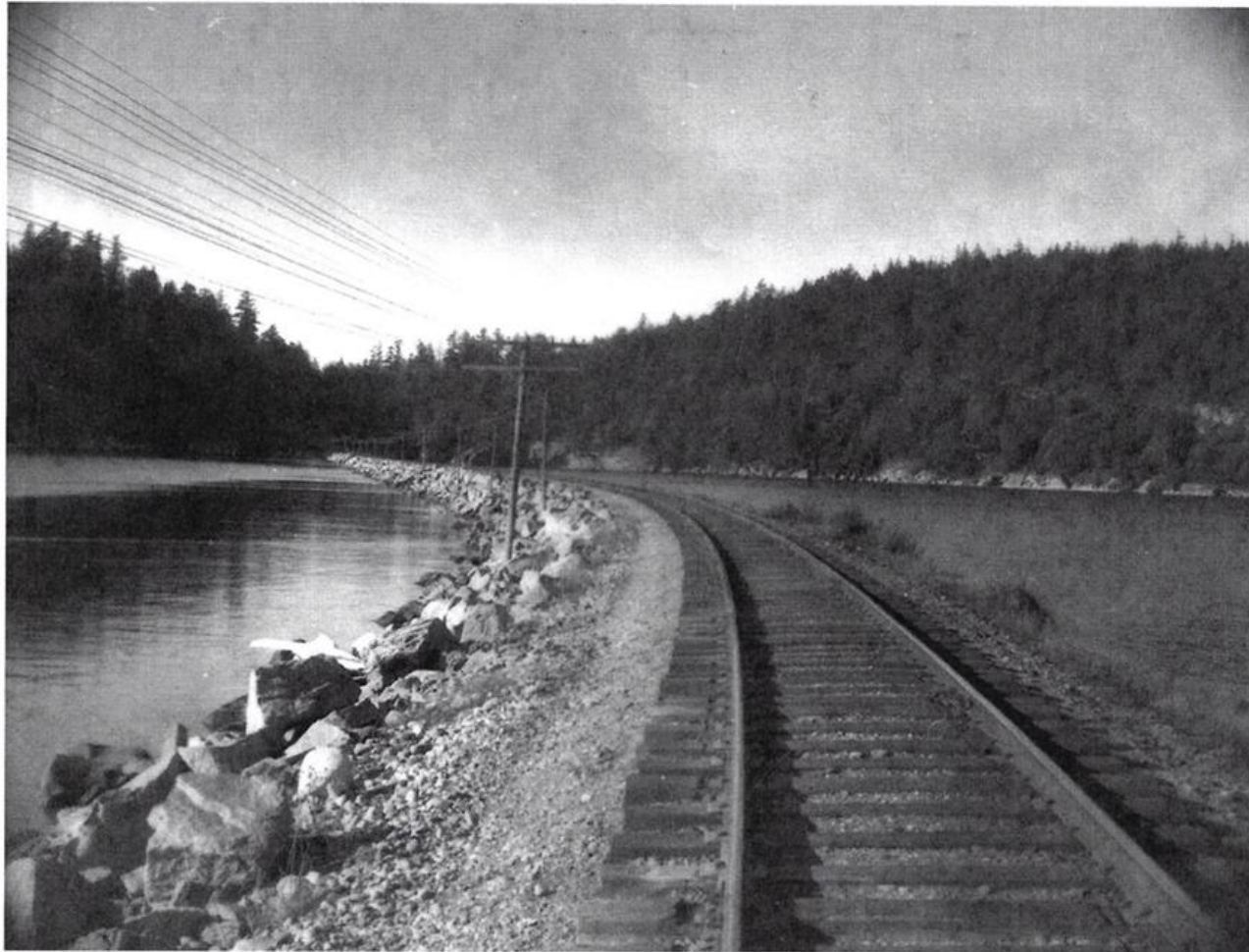
Figure 6: Northwest-facing photograph of the 1920s causeway. Note that this causeway effectively blocks the mouth of the bay. Image taken by Jack Carver, date unknown, and provided courtesy of the Whatcom Museum.
