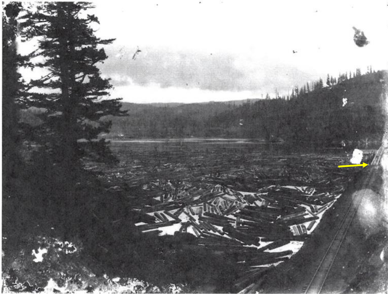
Figure 5: East-facing photograph of Mud Bay with the causeway in the lower right corner, and the position of the 69-m-wide opening indicated with a yellow arrow. The date of this image is unknown, but it was taken after 1920 based on the causeway in the photograph, and is the latest evidence of log-boom storage found for this project. Image courtesy of the Whatcom Museum.
