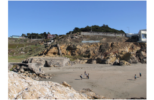
81. Visitor Center to Far Left, Abrupt Edges Revealed
