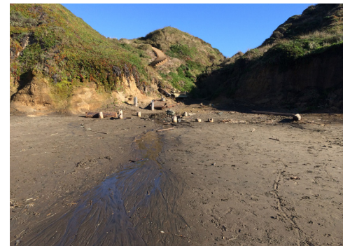
50. Seep Surfacing at Beach
