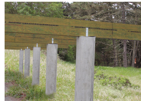
129. Wood and Concrete Set Lightly Into Sand
