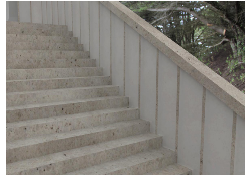
125. Rail Detailing with Infilled Materials
