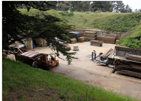
112. Work Yard at Livingston-Springer
