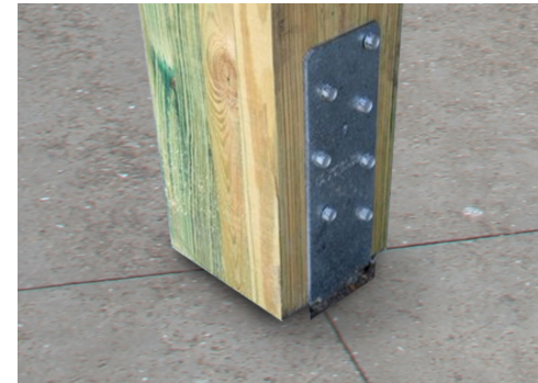
128. Wood Pilings Shackled to Emplacements
