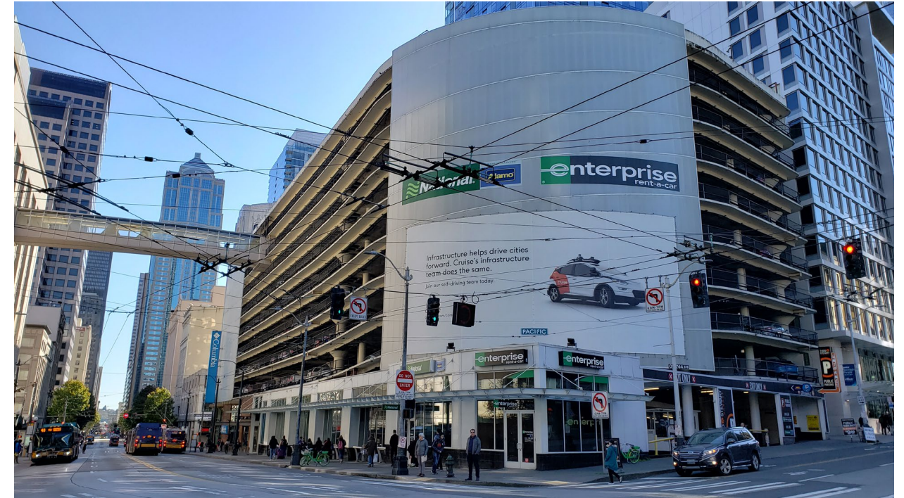
Figure 5.01 Bon Marche Parking Garage, downtown Seattle from Stewart Street and 3rd Avenue.
