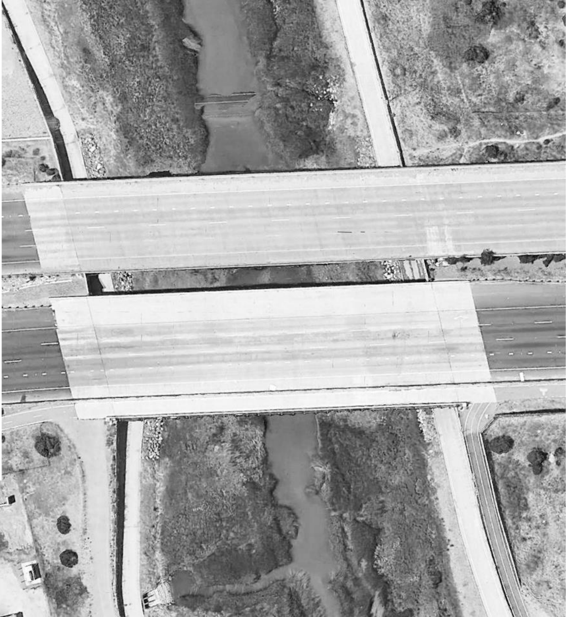
Figure 5.36. Location 3: unsafe and unappealing marginal space underneath the freeway.
