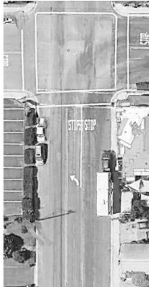
Figure 5.32. Location 1: current wide vehicle lanes and narrow pedestrian walks.
