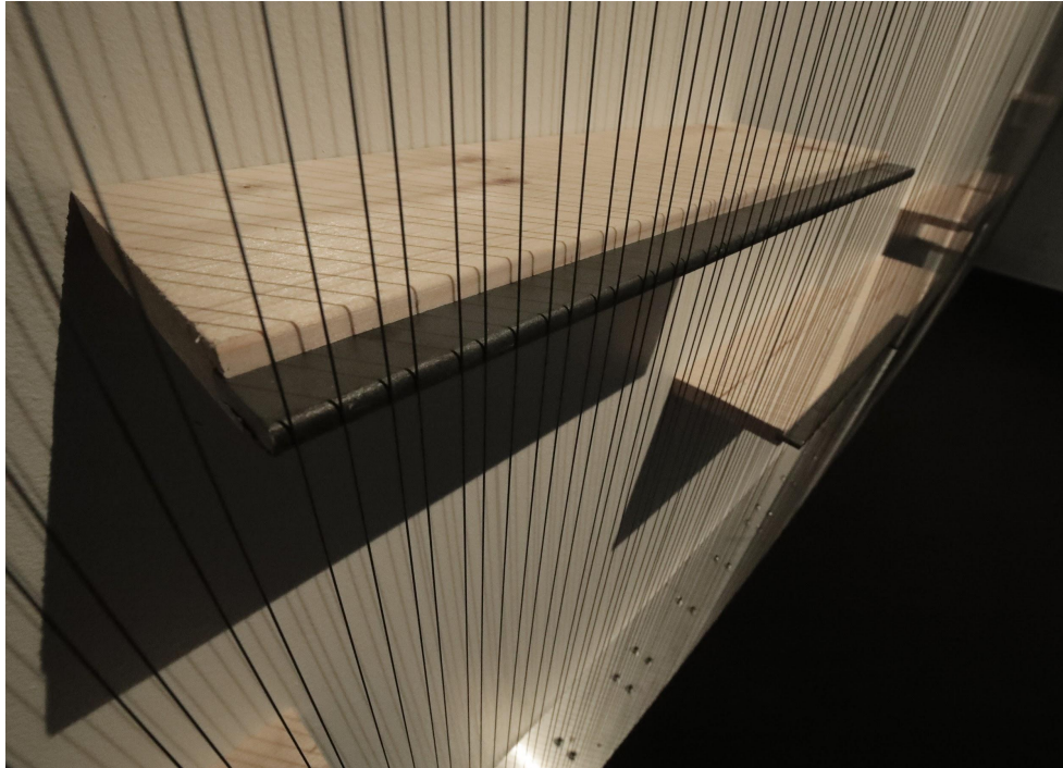
Figure 55 - detail of lower bridges with steel edge
