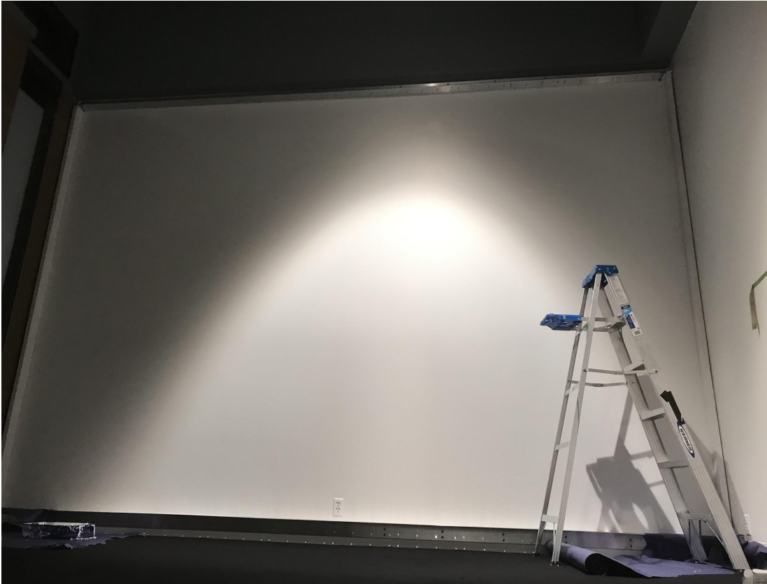
Figure 47 - Large String Array south facing wall with frame installed
