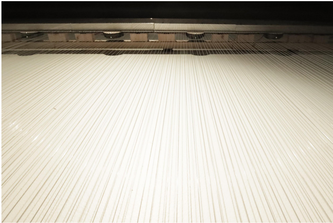
Figure 53 - Looking up at upper bridge with transducers
