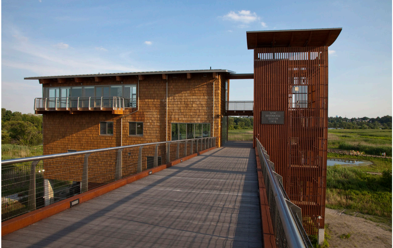
Figure 16 - The naturally ventilated staircase tower stands out from the rest of the structure, while encouraging a spatial connection with the exterior.
