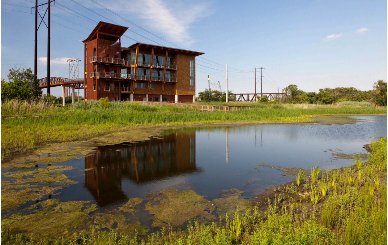
Figure 14 - The transparent facade and the project balconies of the Education Center creates a strong connection with the Christina River marshlands.
