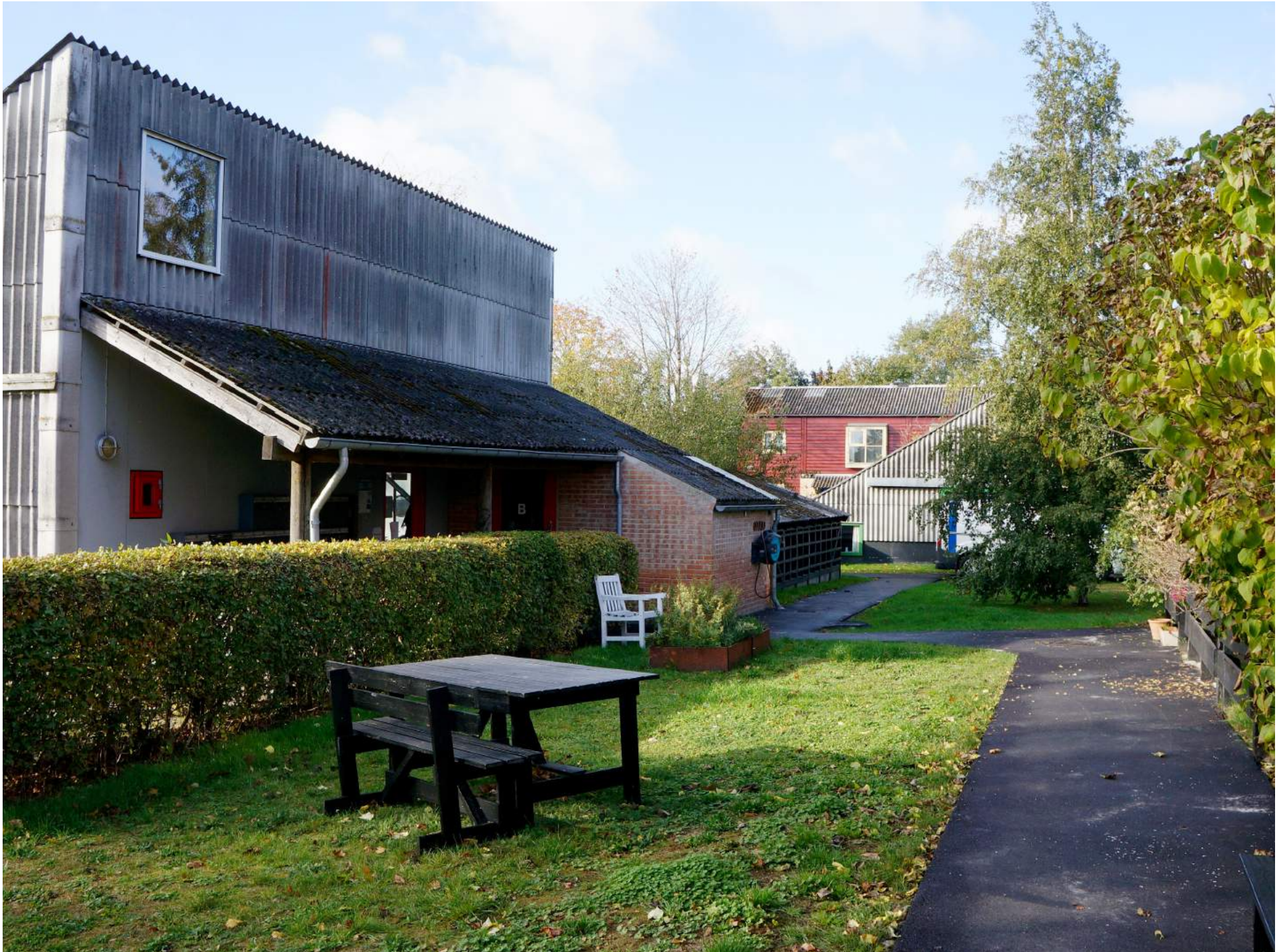
Figure 3-16: Tinggård I Group B common house from the outside. Note unedged asphalt paths and exposed materials including plywood in the common house contributing to the “cheap” look of the architecture.
