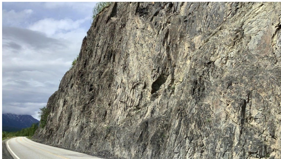
Figure 2.3 Example of carbonaceous mudstone with steeply-dipping bedding at LL71 site.
