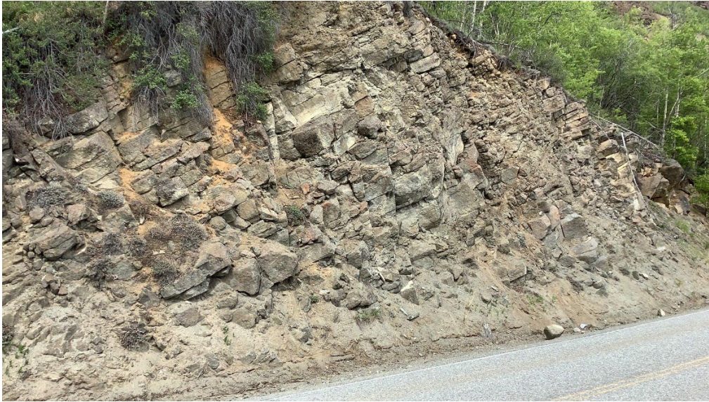
Figure 2.7 Road cut in gabbro at LL 85.5 site.
