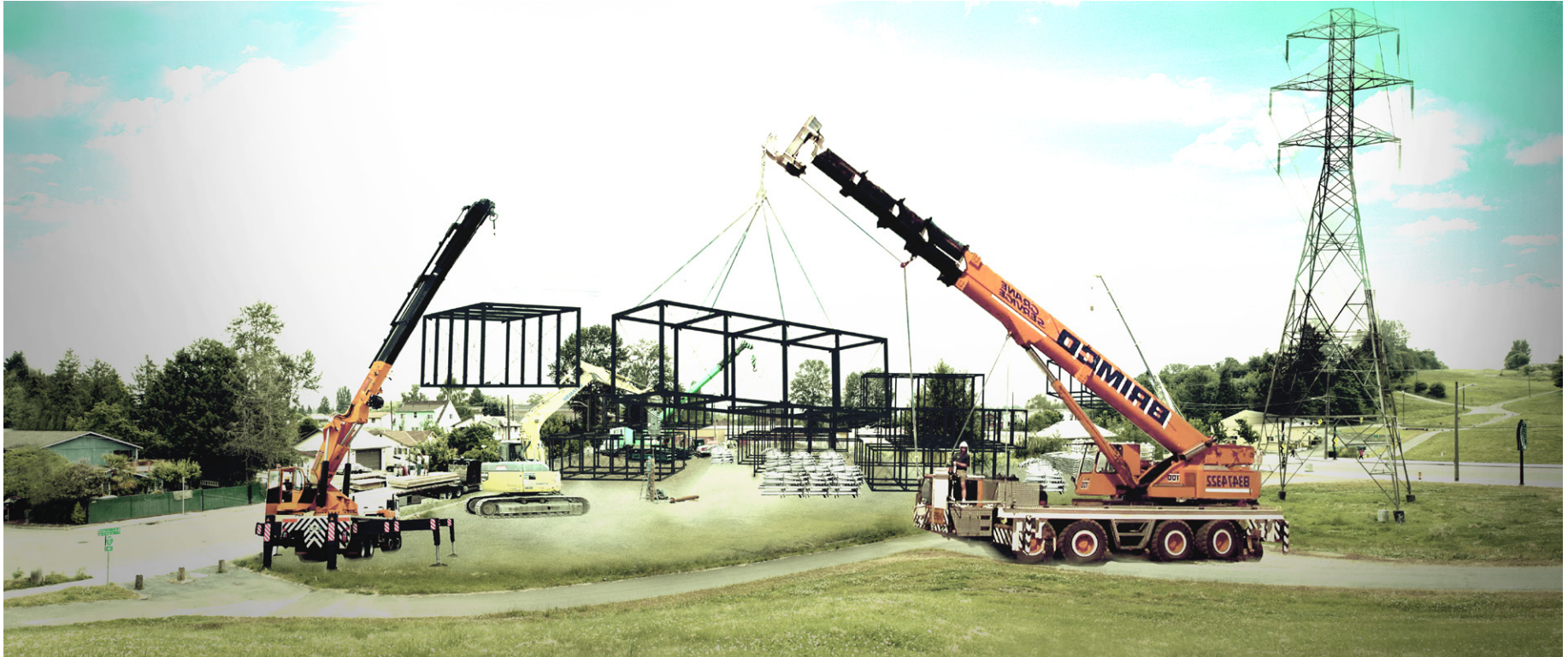
110. Construction perspective from top of berm adjacent to site
