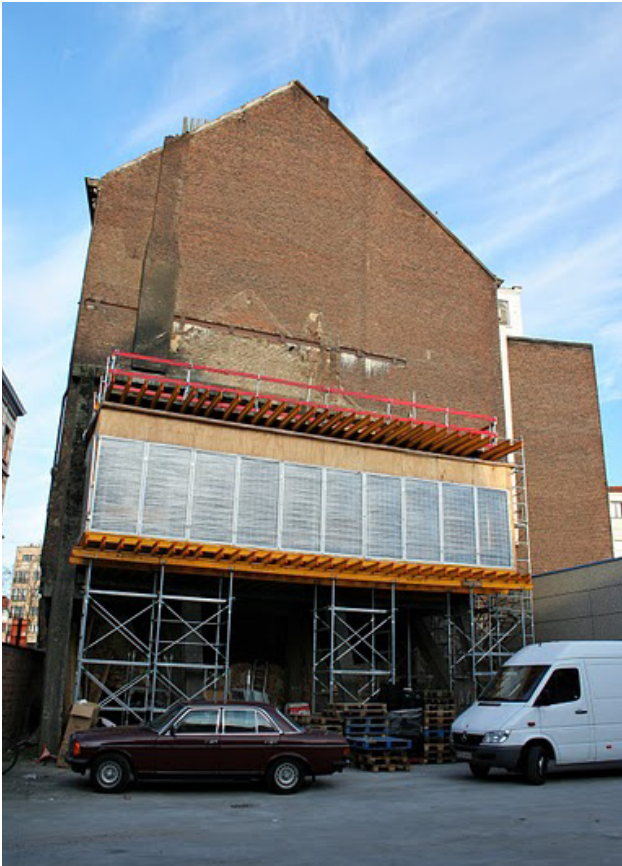
81. RDF 181, Rotor, installation view
