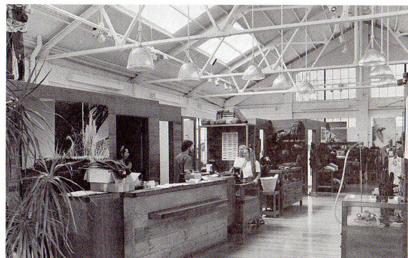
1993 - The 1924 Structure and Skin of the building was so simple and separated from everything else that it remains unchanged seventy years and many tenants later. With its abundant windows and airy steel truss overhead, it makes a cheery shop.
