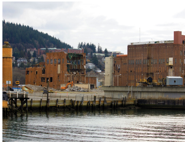
Fig. 7-2 Waterfront Demolition Source: Bellingham Business Journal
