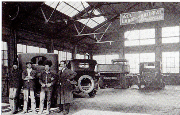
1925 - It was no doubt sometimes too cold and sometimes too hot, but the big clear-span space of the garage had the early-20th-century daylighting that is more appreciated now that it is rare. The metal roof was cheap and effective and still sounds wonderful in the rain.
