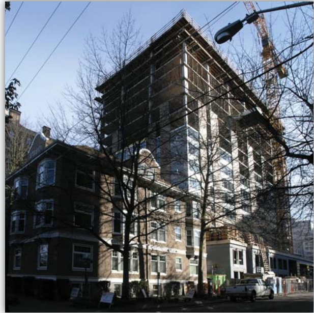
Figure 4.28 – 1200 Madison Street under construction (Nov 2011). Source: Author
