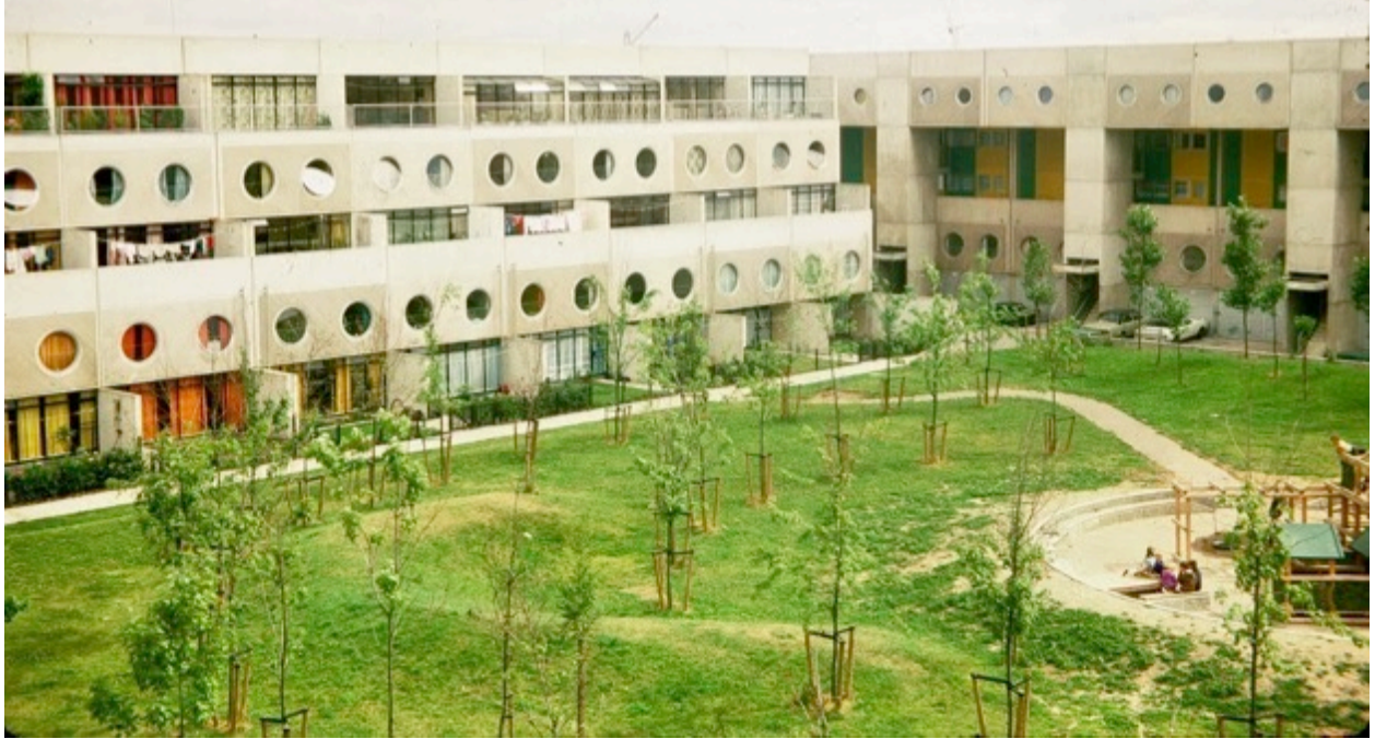
One of Southgate's squares in the mind 1970s. The plastic cladding can be seen at the middle section of the block on the right.
