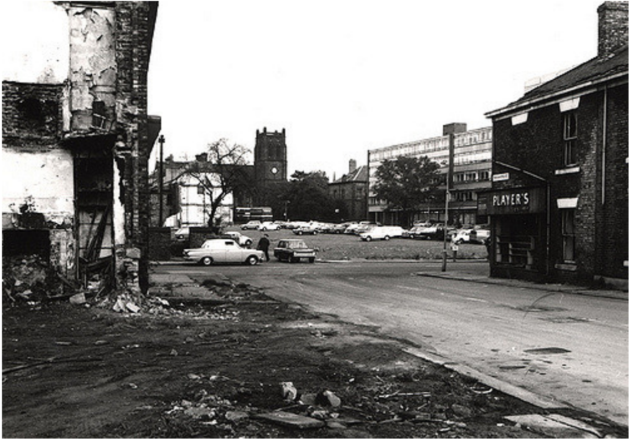
Marianople Street in 1971, after clearance had commenced. Newcastle Libraries, image 042185.
