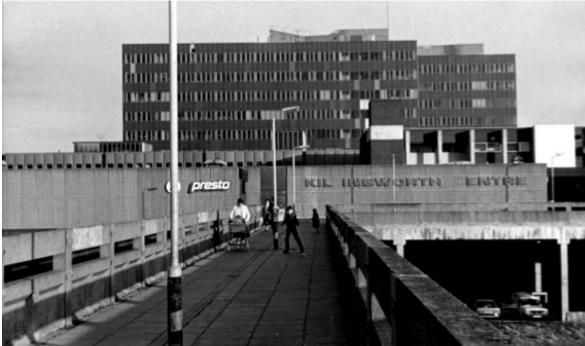
Places of “permanence and security,” part II: the Killingworth Citadel “dominating the landscape” in 1983. In the foreground are the “low bastion” of the shopping mall, and a “street in the sky” leading to the Towers. Deterioration is already evident in the missing sign letters, though the child on roller skates looks happy enough. Photo by Stephen Brain.
