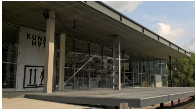
Image 25: Varying columns juxtaposed with each other on the south façade of the Kunsthall. B. Joy
