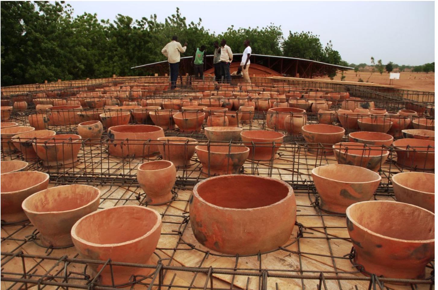
Photograph: roof construction
