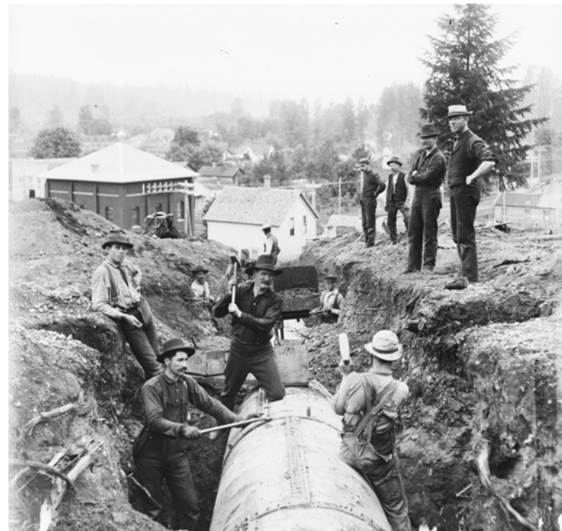
Figure 1.2 Constructing the Cedar River Pipeline, c.1900. Source: Seattle Municipal Archives
