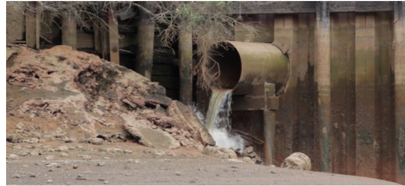
Figure 1.9, A CSO Outfall on the Duwamish River; Photography by Katie Campbell, source: http://www.opb.org/news/article/a-clean-water-act-primer/
