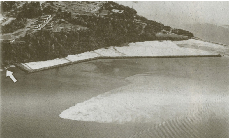
Figure 1.3 The North Trunk Sewer under Construction
