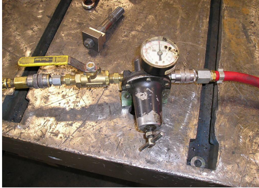
Figure 3.13 Air Pressure Regulator Upstream of Impact Hammer
