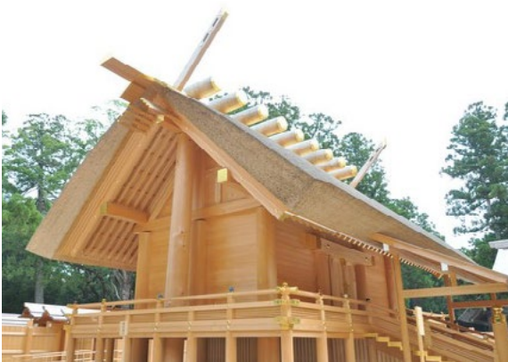
Figure 7: The architectural style of the Jingu Shrine
