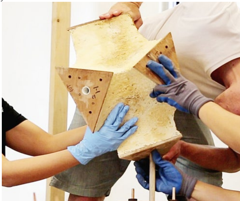
Figure 29: MycoTree component fabrication
