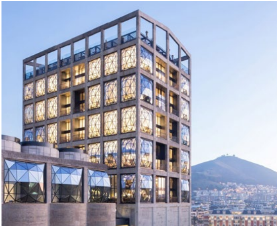
Figure 42: Heatherwick Studio - Zeitz MOCAA art galleries- Cape Town, reuse of a 1920 grain silo
