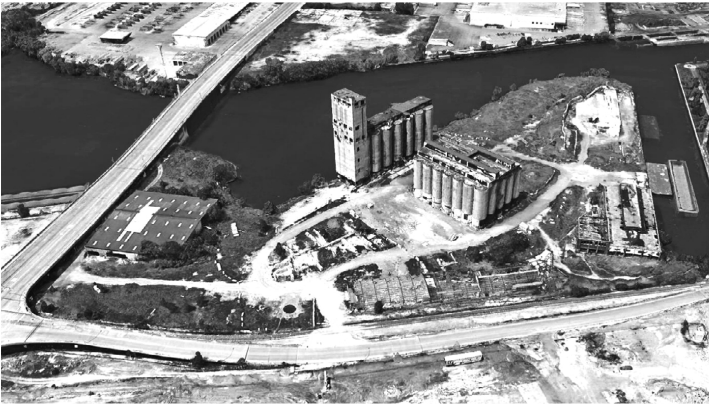
Figure 18: Axon view of the site from Google Earth
