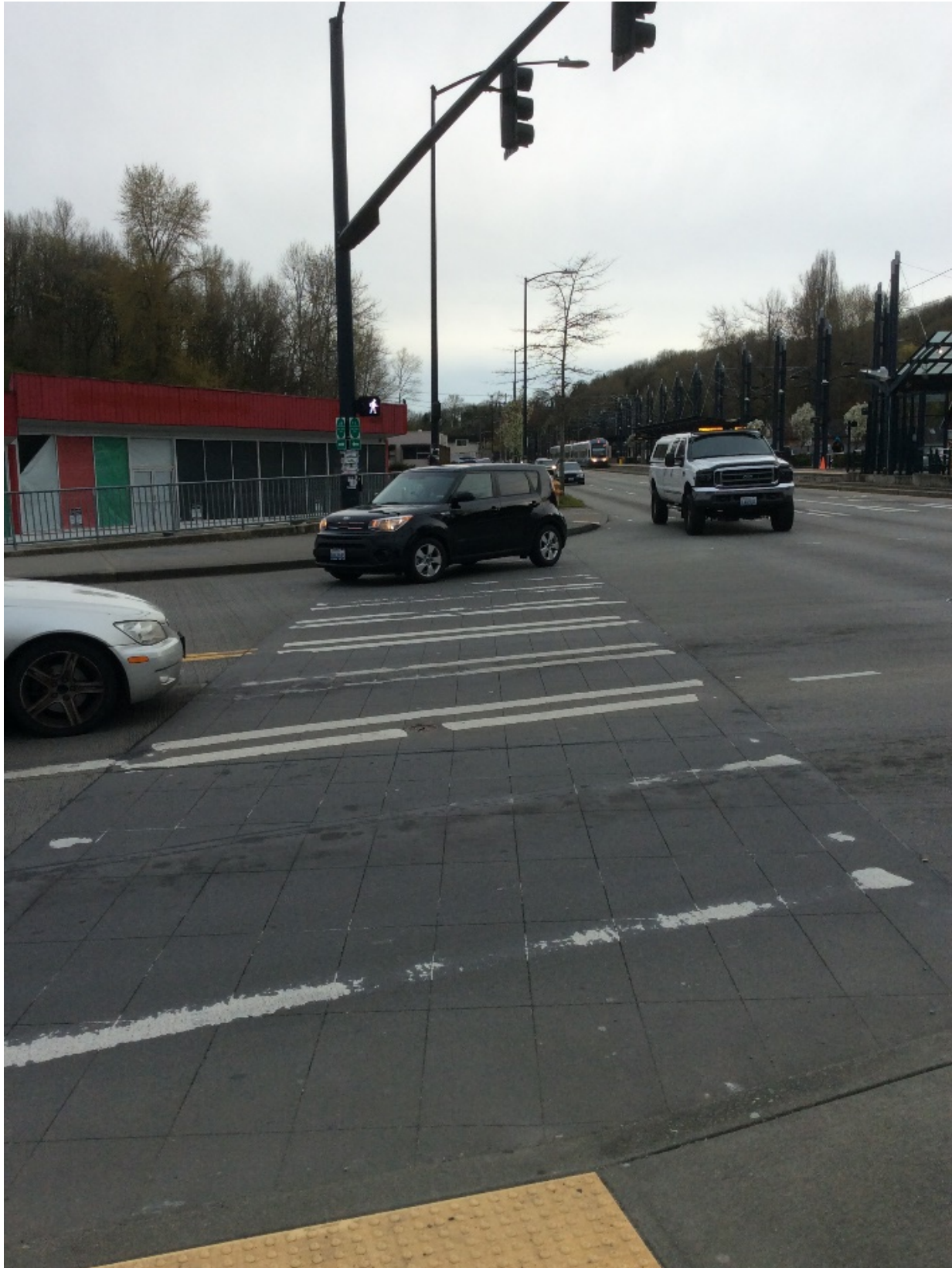
Figure 69: The crosswalk over S Henderson Street near the Rainier Beach Station. (Source: Kaylie Duffy).
