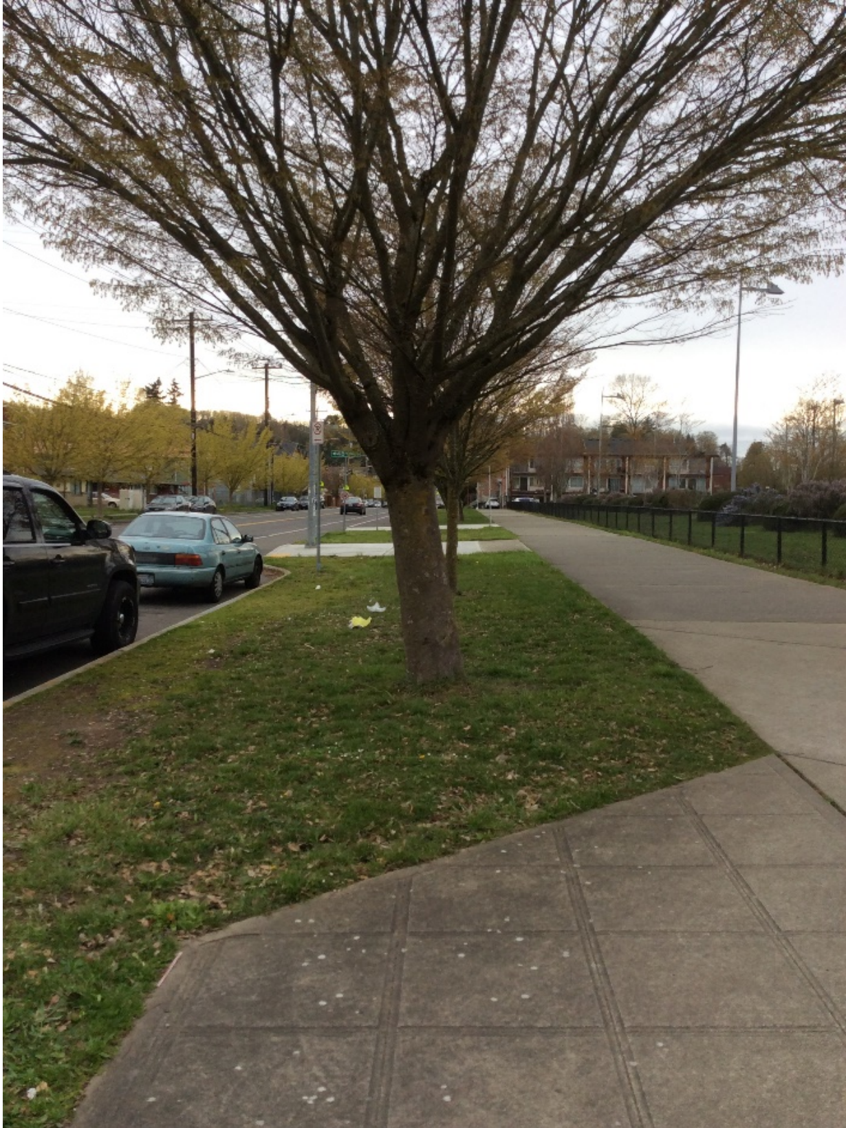
Figure 8: The sidewalks on the north side of S Henderson Street, between 48th Ave S and 46th Ave S, are 12-feet wide and are accompanied by an extra wide planting strip. (Source: Kaylie Duffy).
