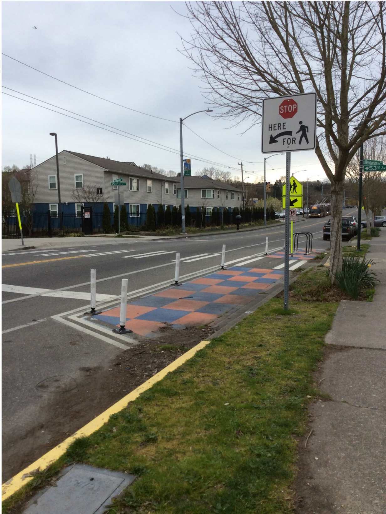
Figure 76: The painted curb bulb on the north side of 53rd Ave S and S Henderson Street. (Source: Kaylie Duffy).
