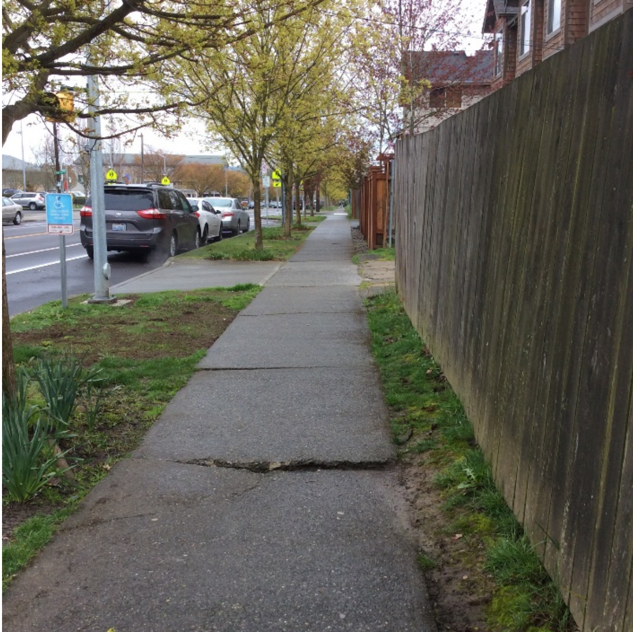
Figure 13: Fences abutting the pedestrian ROW on the south side of S Henderson Street between Renton Ave S and 46th Ave S create an unwelcomed feeling for pedestrians. (Source: Kaylie Duffy).
