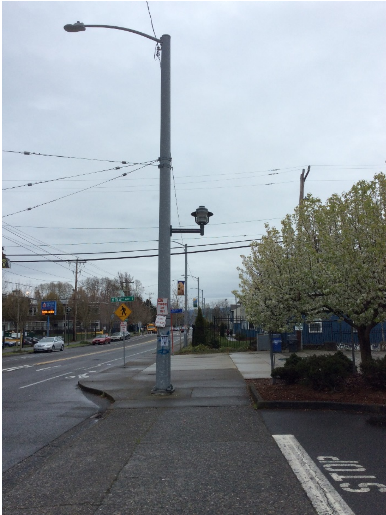
Figure 11: Tall overhead street lights are staggered approximately every 125 to 150-feet over the length of the S Henderson Street. Shorter, more human scale lights are attached to the larger light poles in some locations. (Source: Kaylie Duffy).
