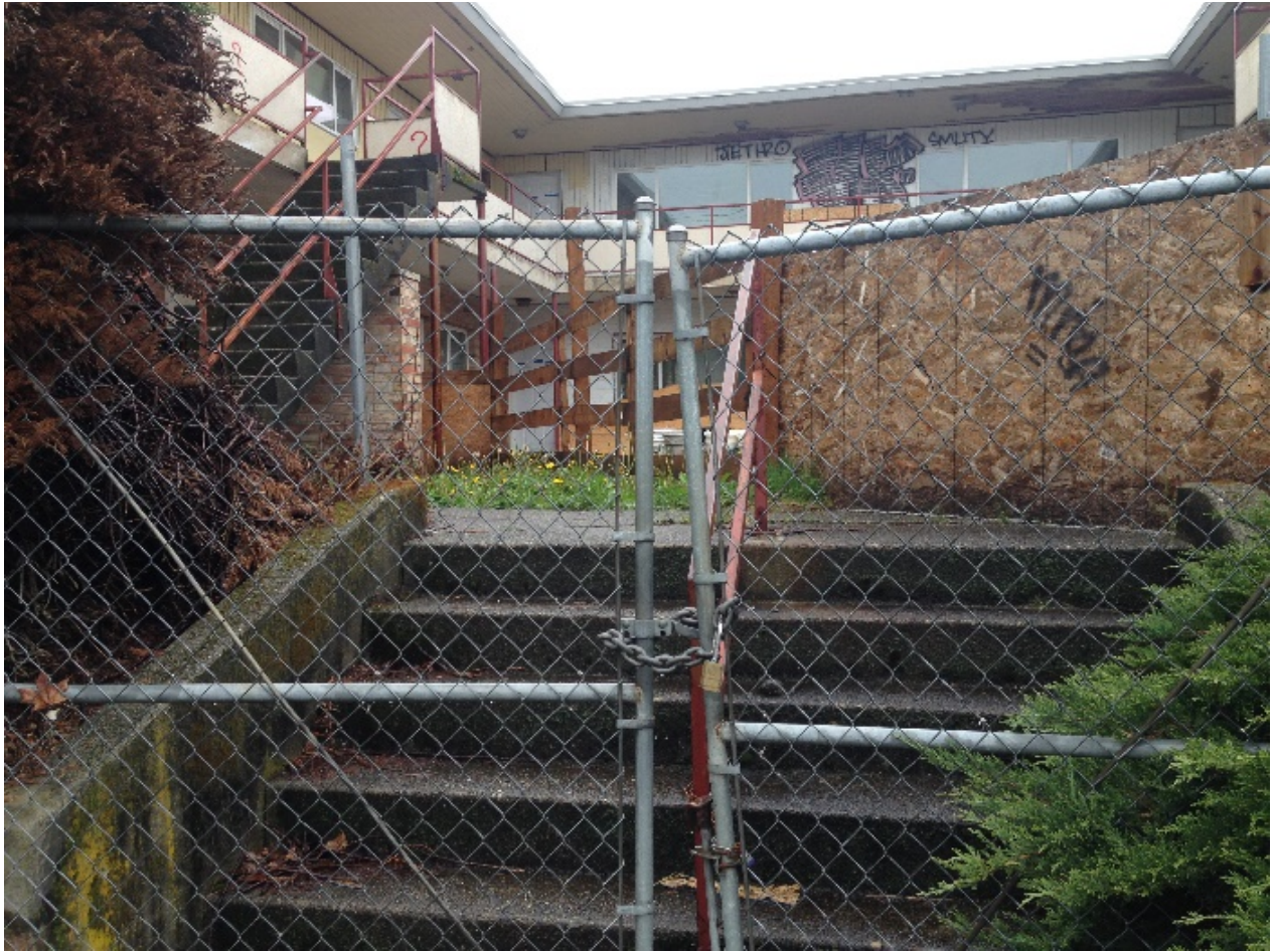
Figure 43: The vacant apartment building on the north side of S Henderson Street, between 46th Ave S and Renton Ave S is unwelcoming and inactivated. (Source: Kaylie Duffy).
