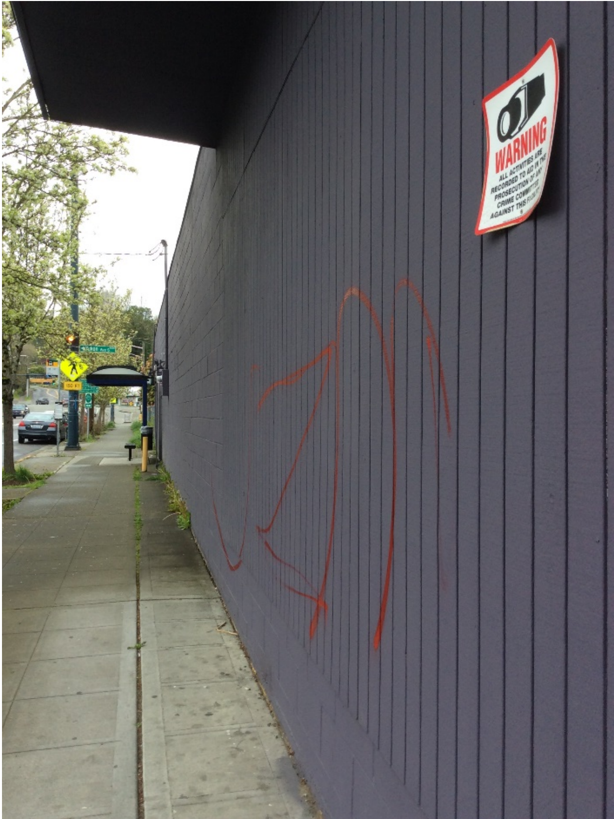
Figure 47: Building awnings, such as the one at the northwest corner of Renton Ave S and S Henderson Street, provide shelter from inclement weather. (Source: Kaylie Duffy).
