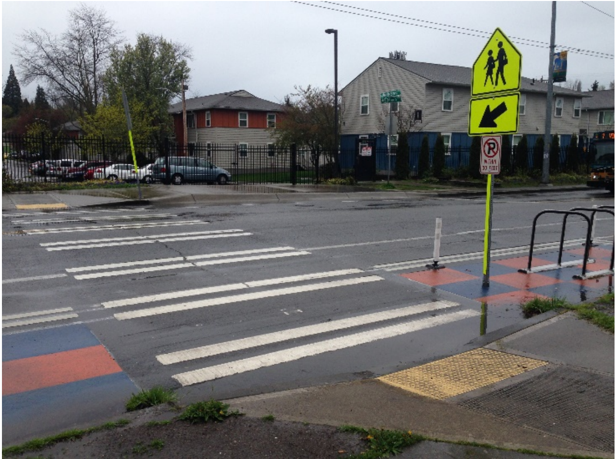
Figure 59: In 2016, SDOT finished construction on a Safe Routes to Schools project by installing a painted curb bulb at S Henderson St and 53rd Ave S near the Rainier Beach High School. (Source: Kaylie Duffy).
