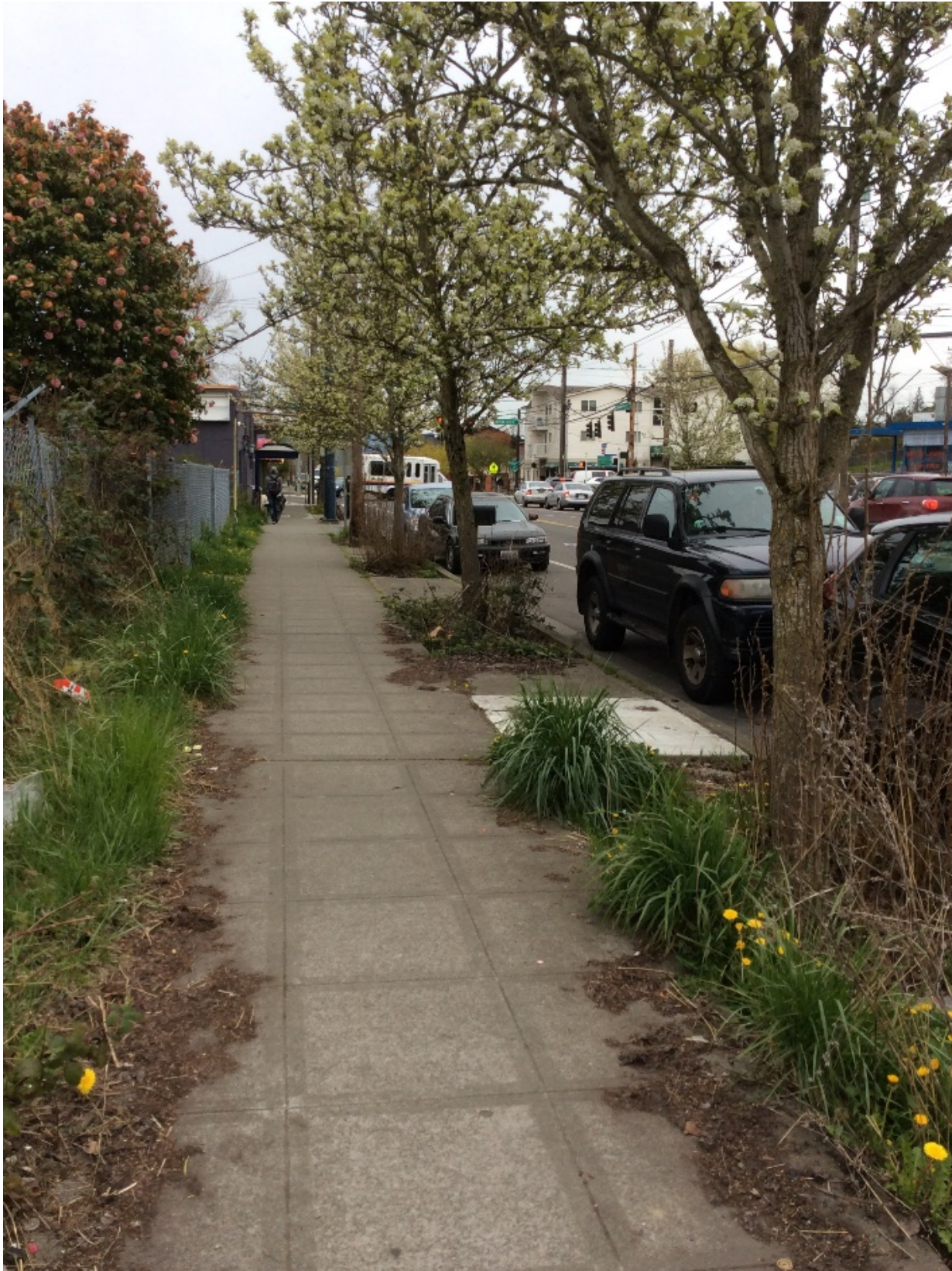
Figure 9: This sidewalk is on the north side of S Henderson Street, between Renton Ave S and Chief Sealth Trail. While the sidewalk is 6-feet wide, the overgrown planting strip and yard edges make it appear smaller. (Source: Kaylie Duffy).
