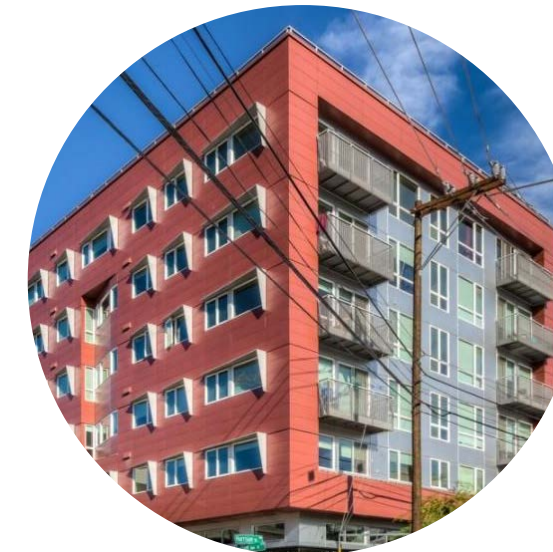
5.5 Cascade Apartment Building | Image source: rent.com
