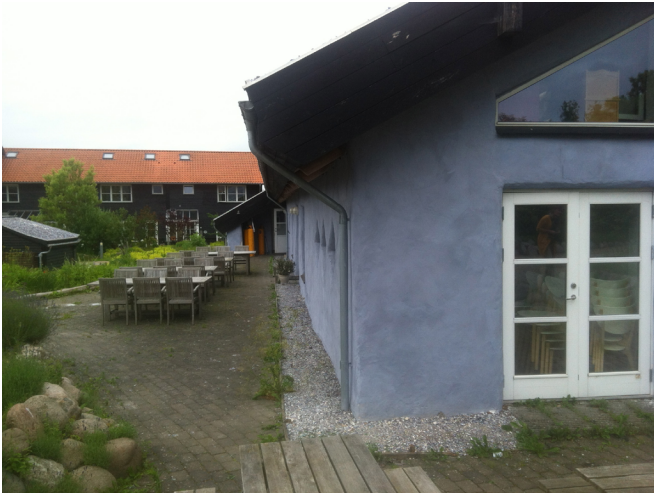
Fig. 14: Exterior view of the Munksøgård common house, built with straw bale and local timber. (image by the author)
