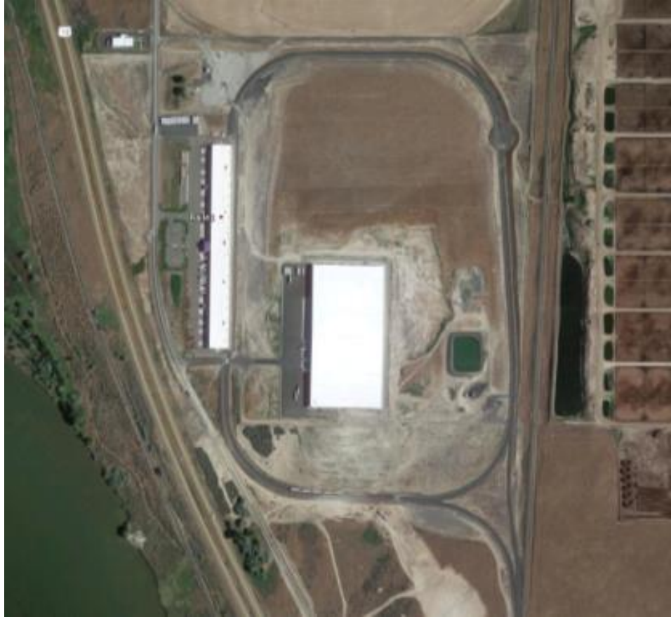
Figure 6.9 Aerial View of Railex Facility in Wallula, WA. Loop Track Allows 19 Cars to Enter the Building on the Left for Loading. Photo from Google maps
