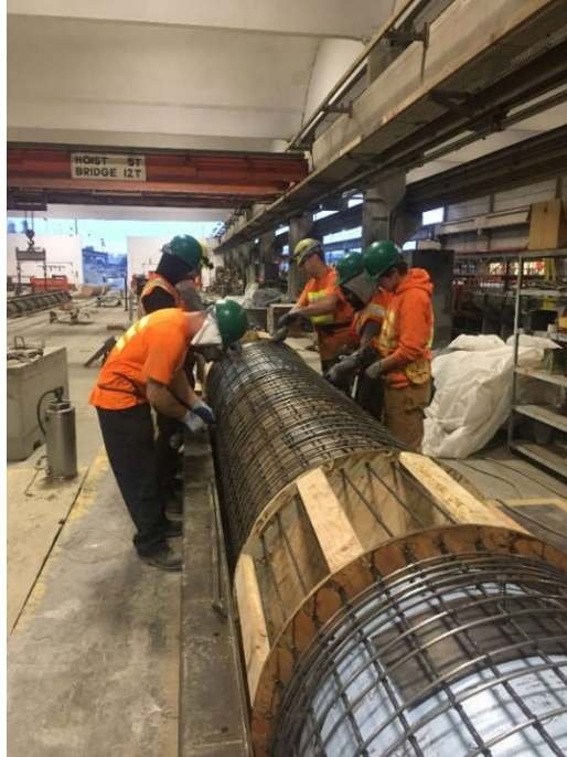
Figure 7-8. Column reinforcement being prepared for casting at Concrete Technology Corporation
