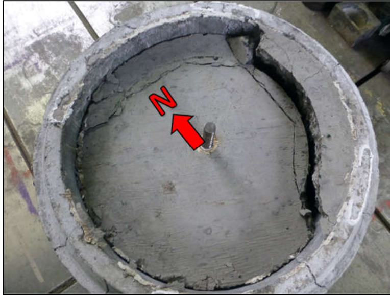
Figure 5-14. Plan View of Test 6-ep24-cr at end of test showing "punching" failure on east side of specimen
