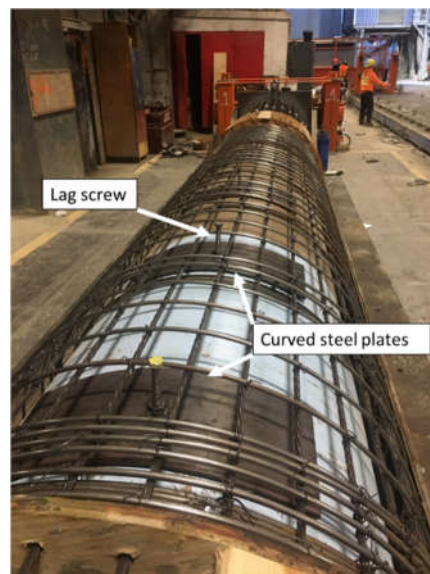
Figure 7-11. Hold-down plates used for sonotube during casting
