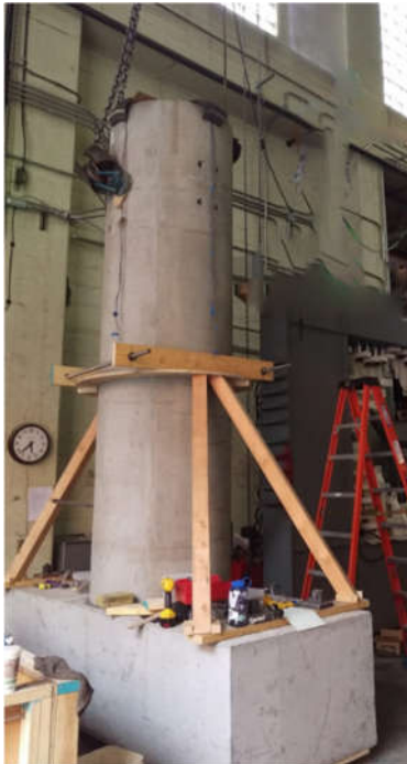
Figure 7-19. Column braced on top of cap beam
