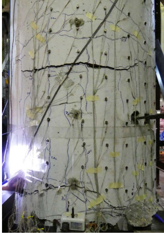
Figure 8-12. Very wide crack on north face, Series 8
