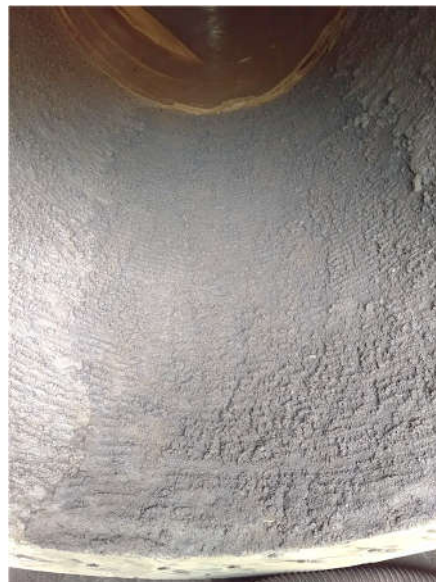
Figure 7-18. Inner surface of column roughened with epoxy mortar
