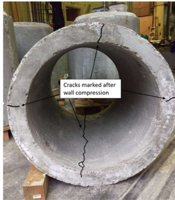
Figure 4-9. Longitudinal cracks - Specimen ep24-cr
