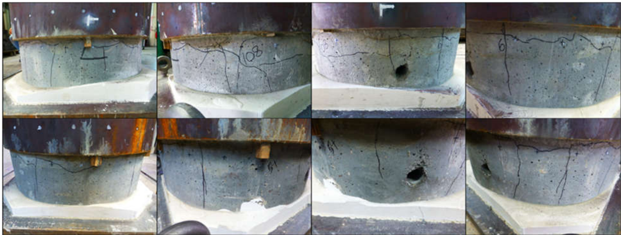
Figure 5-19. Crack formation at end of testing for Test ep24s4-1 (L-R: N-NW-W-SW; S-SE-E-NE)
