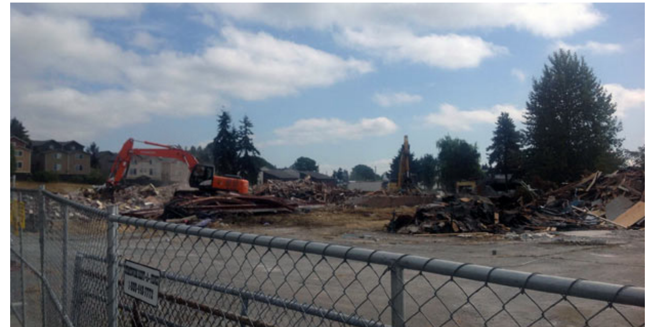
Figure 107: Woodrow Wilson School demolition in 2015. (Robertson 2015)
