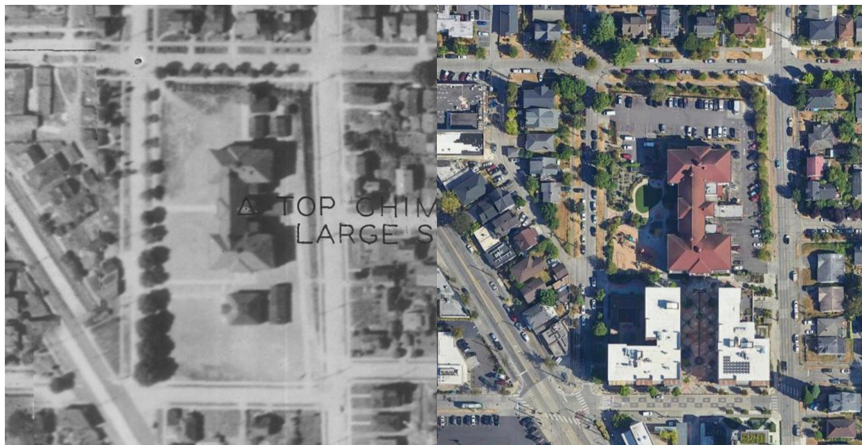
Figure 57: Aerial map of Beacon Hill School in 1936. (Historic Aerials 1936)
