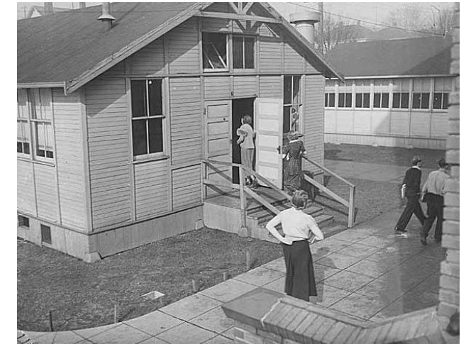
Figure 22: Portable building in use at Ballard High School (Nelson 1988)
