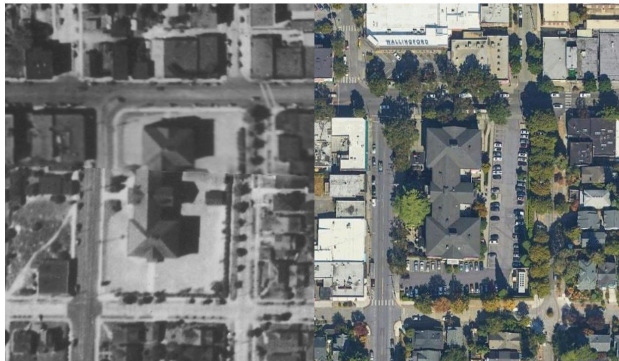
Figure 36: Interlake School aerial 1936. (Historic Aerials 2023)
