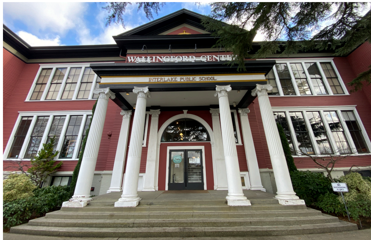
Figure 34: West face elevation of Interlake School. (Photo from author 2021)
