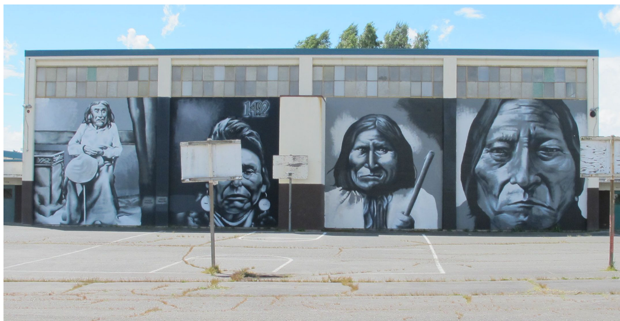
Figure 93: Woodrow Wilson School, gymnasium exterior, photographed in 2013. (Johnson and Mirro 2013)
