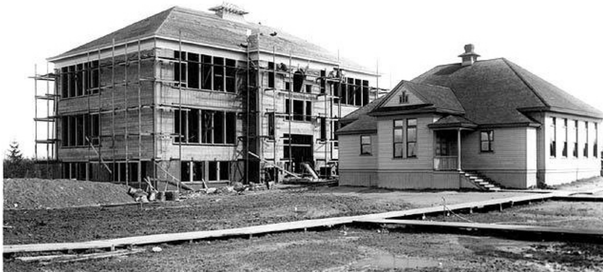
Figure 61: Beacon Hill School under construction in 1904. (Asahel Curtis Collection CUR328)
