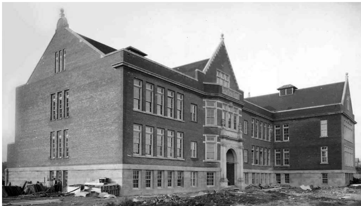
Figure 76: Colman, viewed looking northwest, nearing completion in 1909. Note the flat facade (south) intended for a further classroom-wing. (Thompson and Marr 2001)
