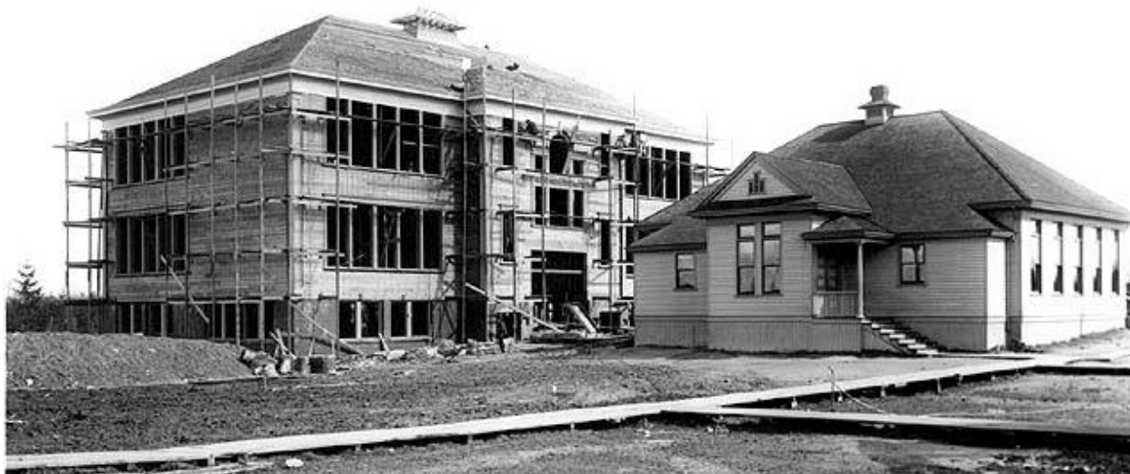
Figure 21: Beacon Hill School, a wood-frame model-school, under construction in 1904 prior to expansion. (MOHAI)
