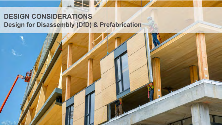
Figure 25. Prefabricated wall panel construction.
