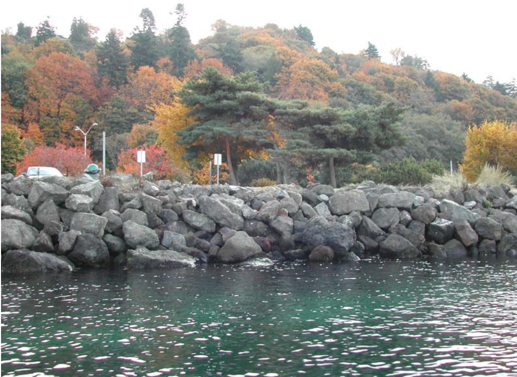
Figure 8. Shoreline retained with rip-rap.
