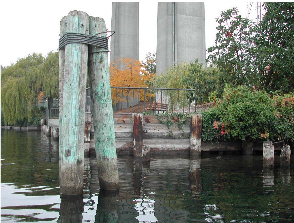
Figure 10. Shoreline retained with a wood bulkhead.
