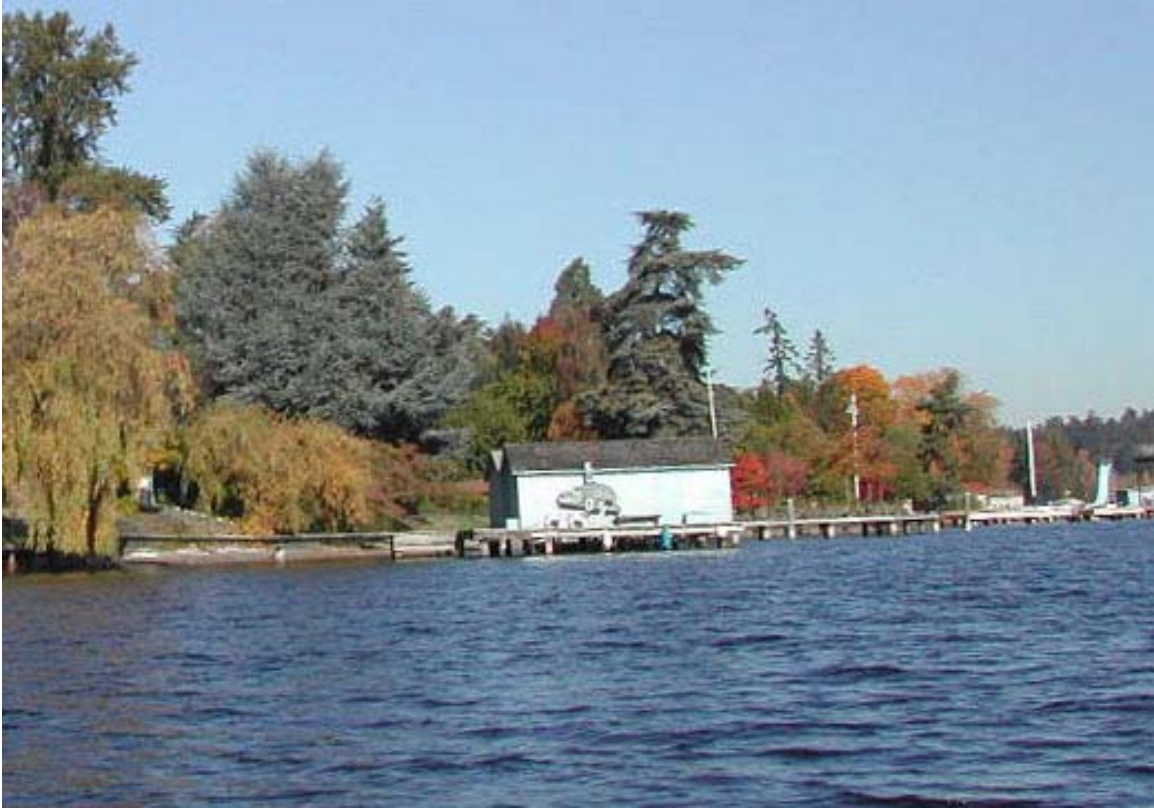
Figure 7. Dock with attached building.
