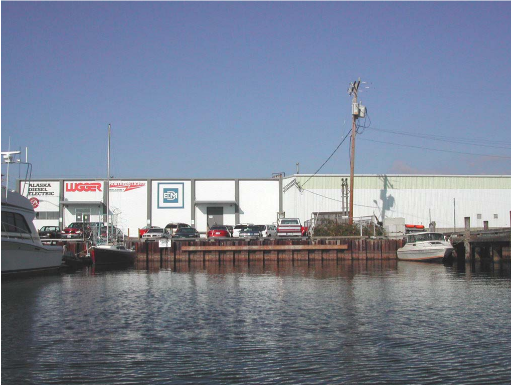
Figure 9. Shoreline retained with a steel bulkhead.
