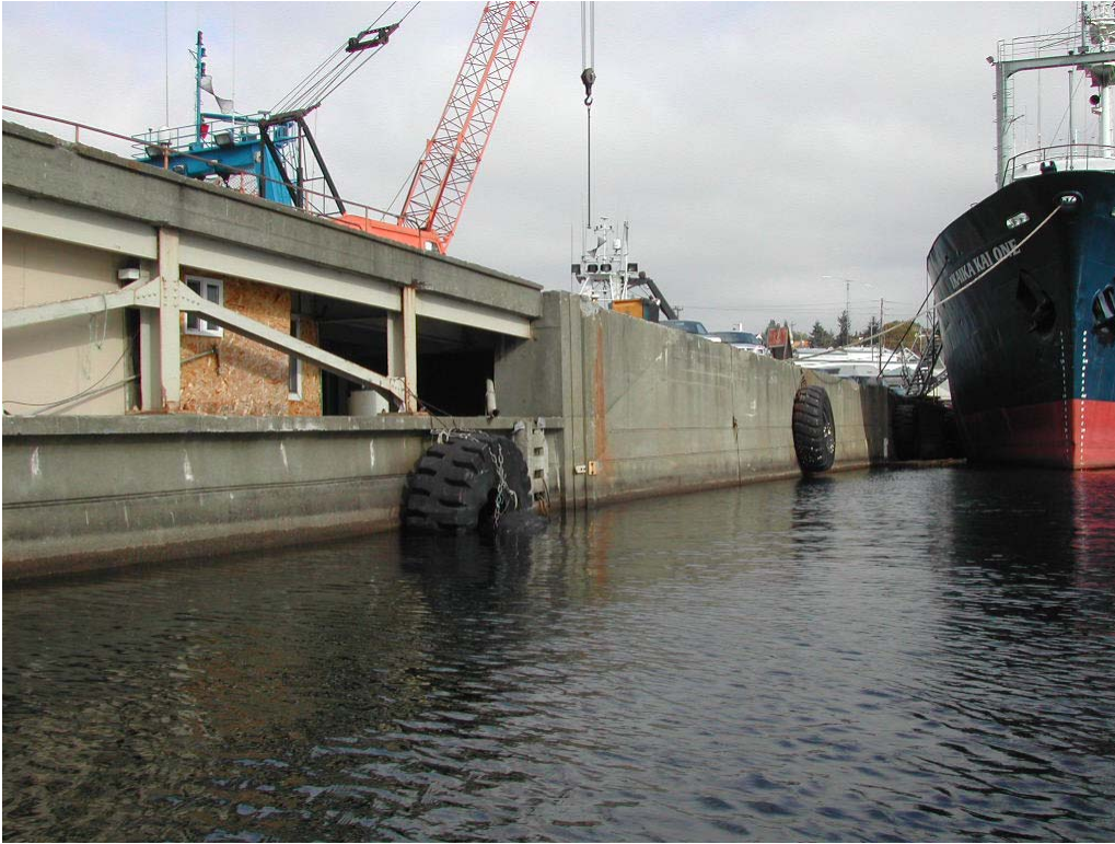
Figure 11. Shoreline retained with a concrete bulkhead.
