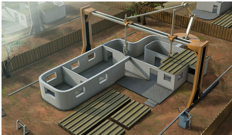
Fig. 133: Construction Method of Contour Crafting - a Company that is Conducting R&D to Build in Outerspace
