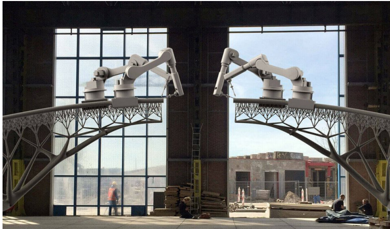
Fig. 132: World's First Digitally Fabricated Bridge - The Bridge that Built Itself.
