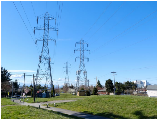
Fig. 1-6: The power line towers on the trail
