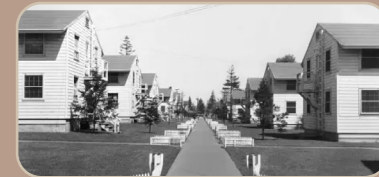
Fort Lawton's barracks after they were constructed in 1942.
