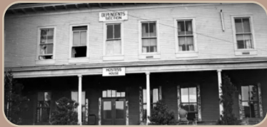
Fort Lawton Hostess House.
