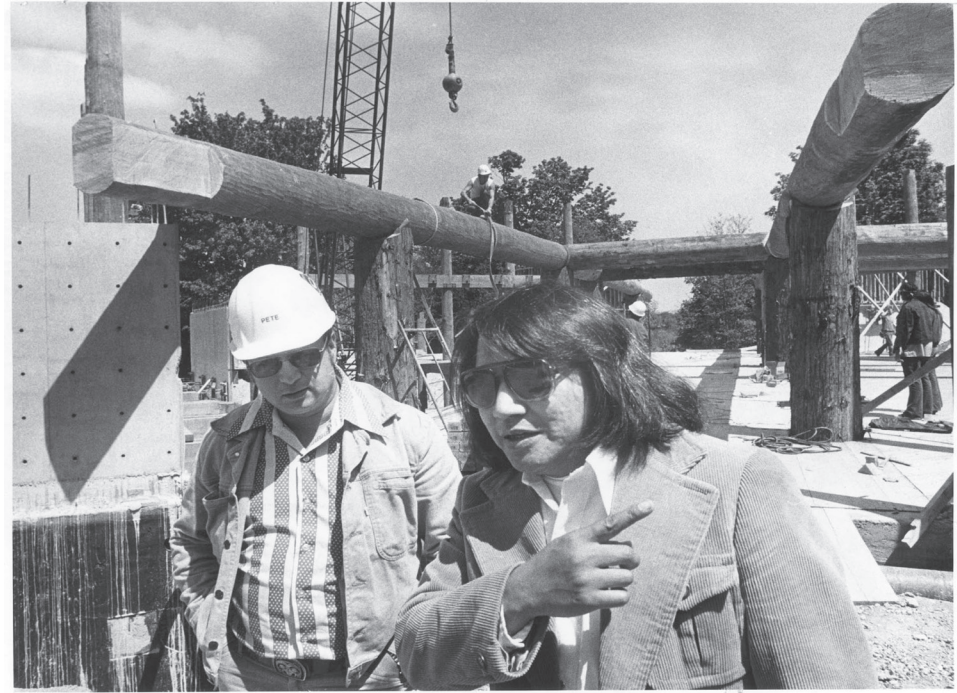
Bernie Whitebear and Pete Schnurman (1938-2020), lawyer for United Indians of All Tribes Foundation, at the construction site of Daybreak Star Indian Cultural Center, 1976.
