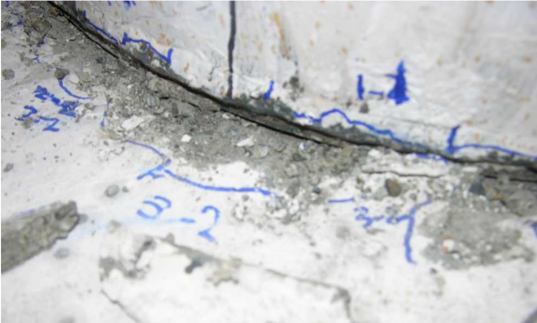
Figure C.10 Footing fillet-spalling.
