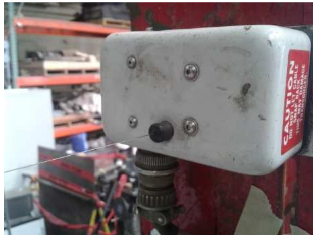
Figure 3.9 A string potentiometer attached to the instrumentation tower.
