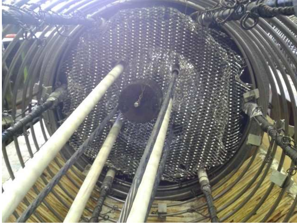
Figure D.2 Dividing mesh used to separate the HyFRC and conventional concrete pours (Image before casting).
