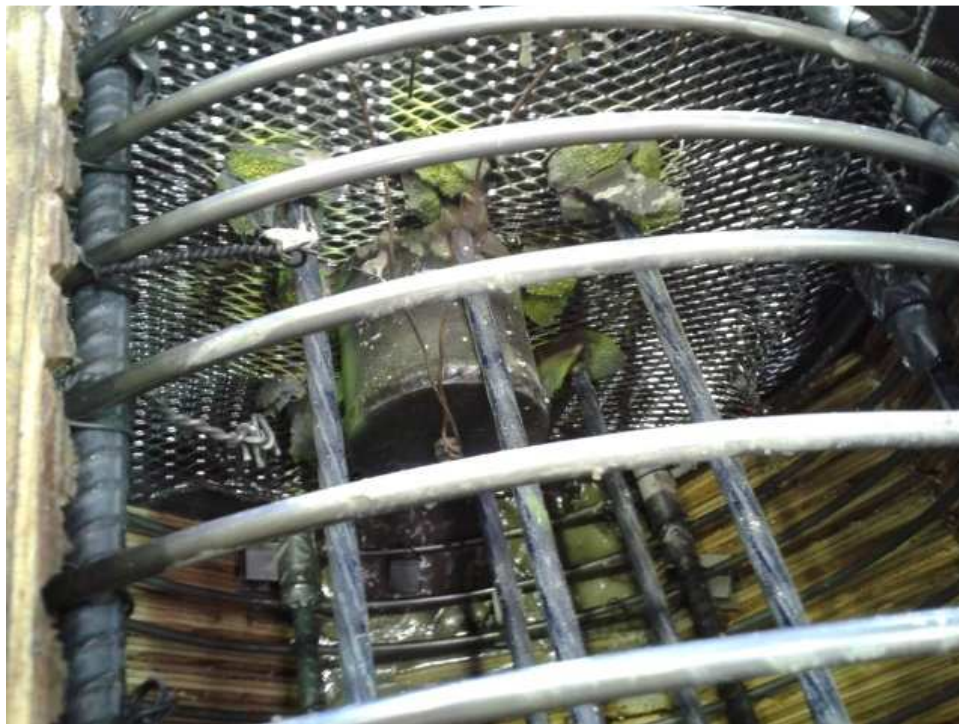
Figure D.3 Dividing mesh used to separate the HyFRC and conventional concrete pours. (Image after casting).
