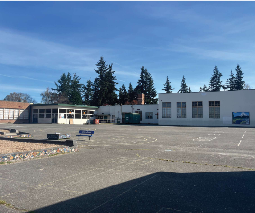
Fig 7.5: Lower grade playground looking toward covered area and asphalt area.
