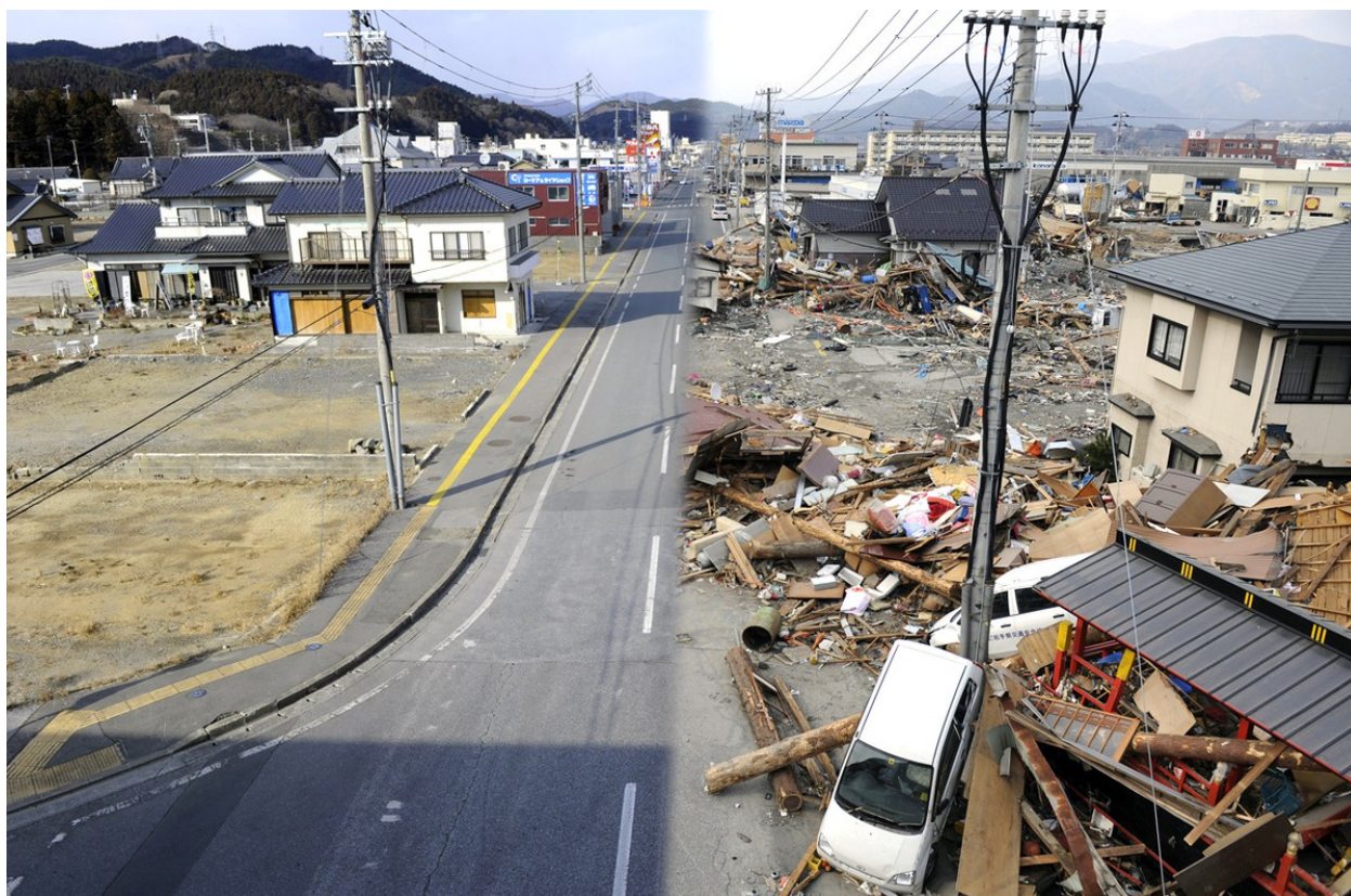
Fig. 1.1. Tsunami-driven debris-field impacts on Ofunato, Japan. Debris-field impact on a street in Ofunato, Japan, as a result of the Tohoku 2011 earthquake and tsunami. (Left) A street in Ofunato following post-disaster debris-field clean-up, taken January 15, 2012. (Right) The same street 3-days after the tsunami, taken March 14, 2011. Photographs courtesy of Toshifumi Kitamura / AFP.
