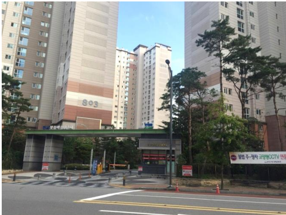
Figure 3-16. A vehicle control system at the entrance of Complex H (source: author)
