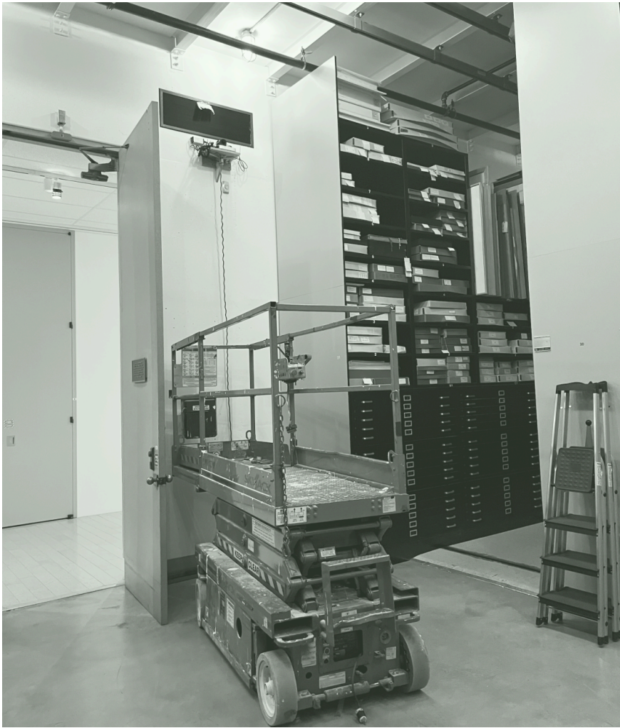
Figure 18. above, installation high on the wall in the Douglas Vault
