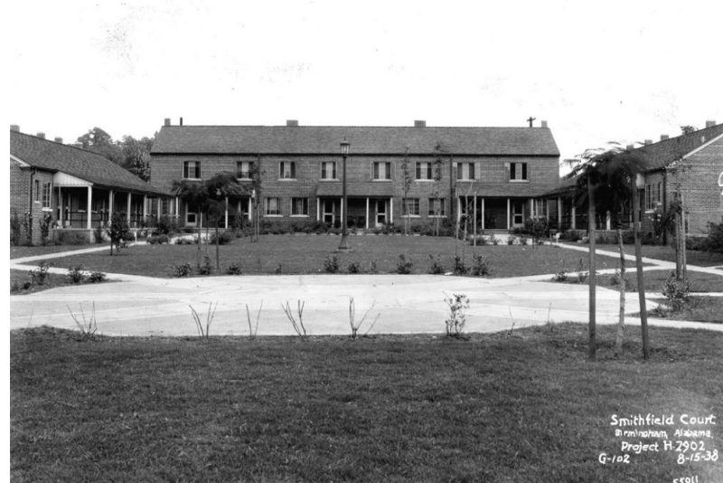
fig. 37 and 38. Typical urban renewal construction in Birmingham.
