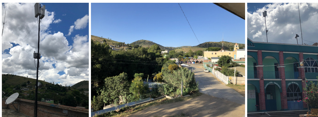
Figure 6.1: From left to right: the trial LTE hardware, the view of the centro in Santa Inés, and the town hall and community telecom office.
