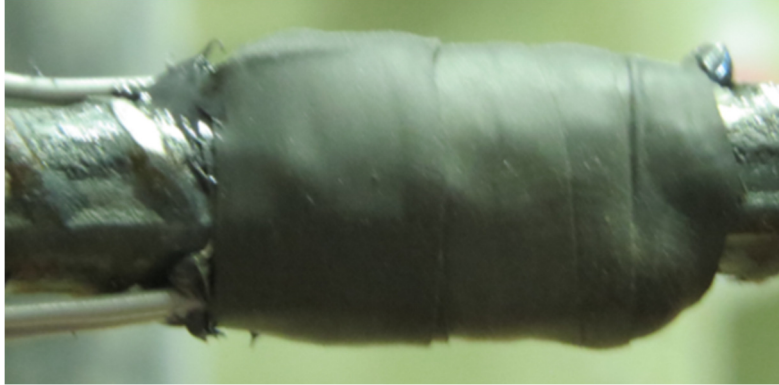
Figure E.3 Waterproof coating applied to strain gauge and folded over lead wires.
