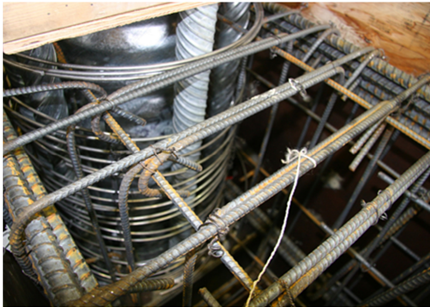
Figure D.10 Cap beam ductwork.
