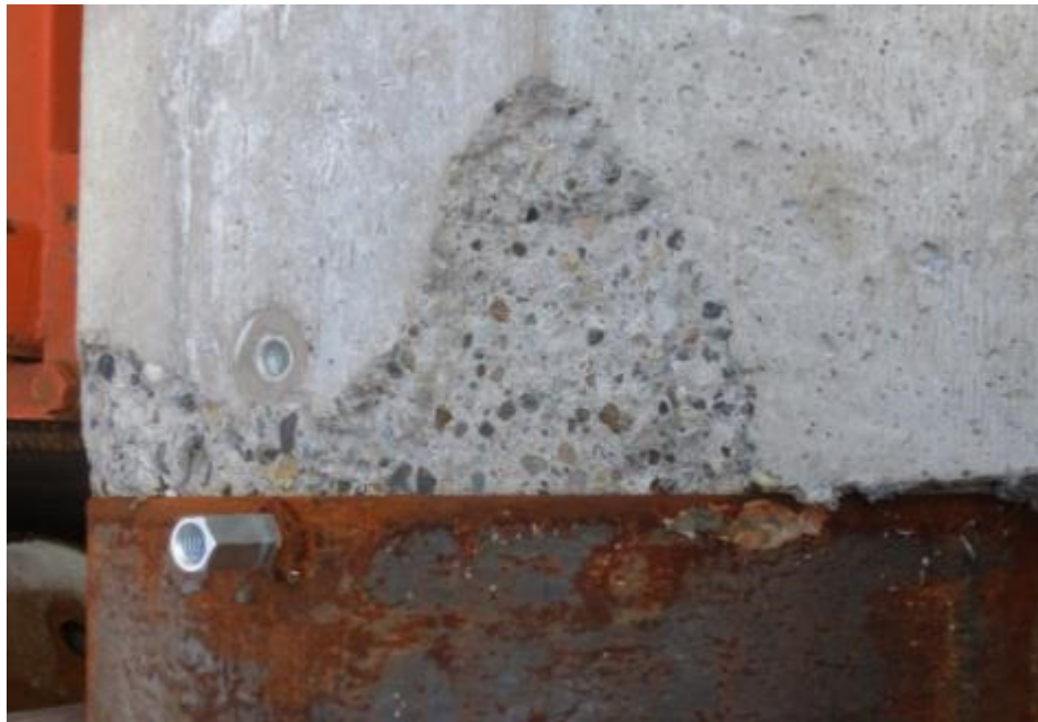
Figure 4.6 Corner spalling of PreT-SF-ROCK specimen.
