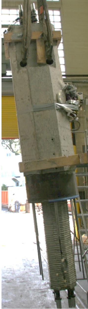
Figure D.6 Crane lift of cast column.
