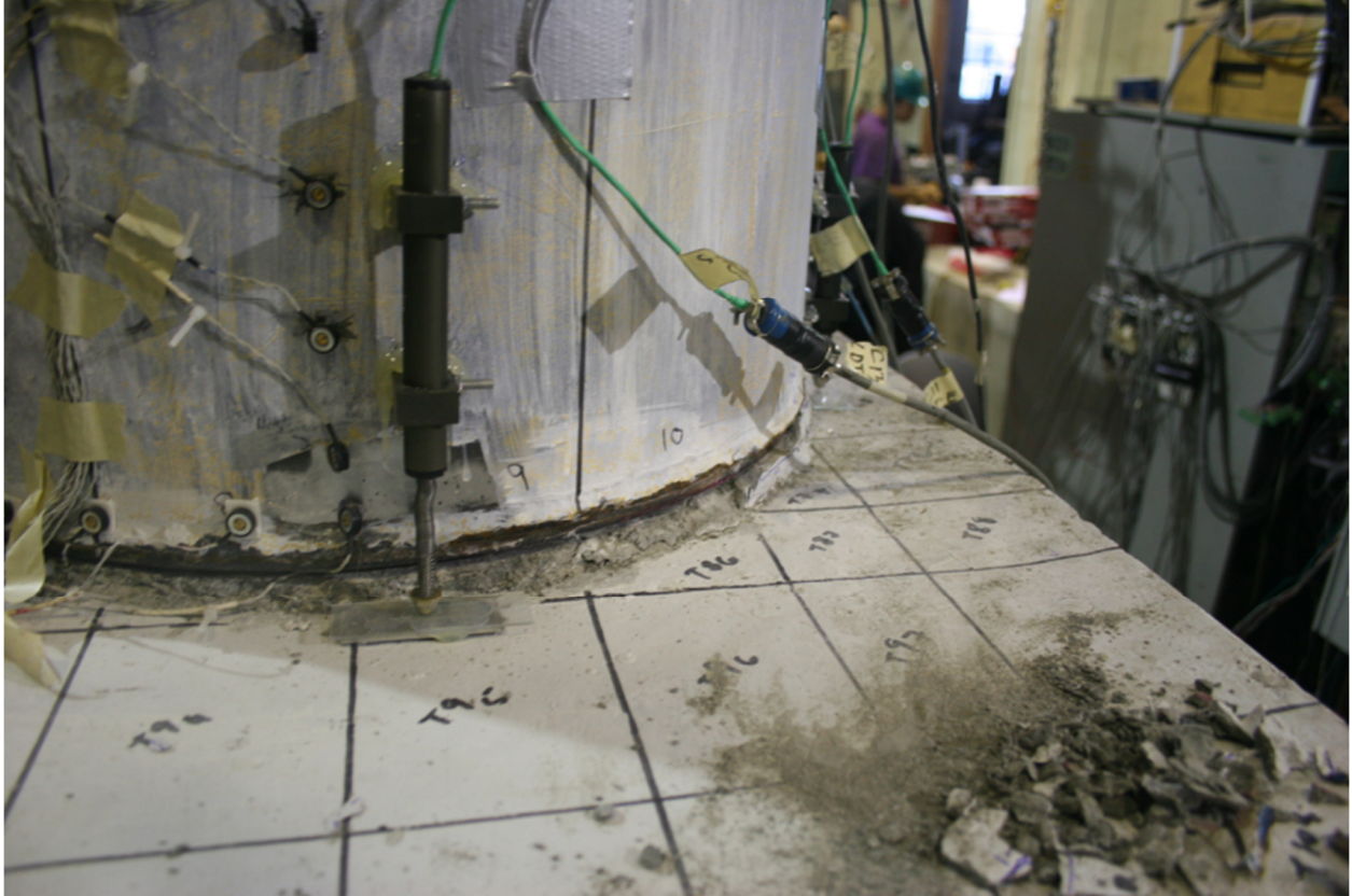
Figure C.5 Grout pad at end of test.
