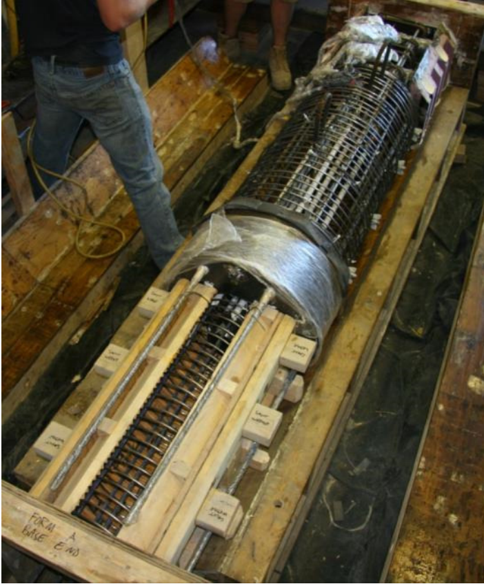
Figure D.1 Column cage and formwork (isometric).
