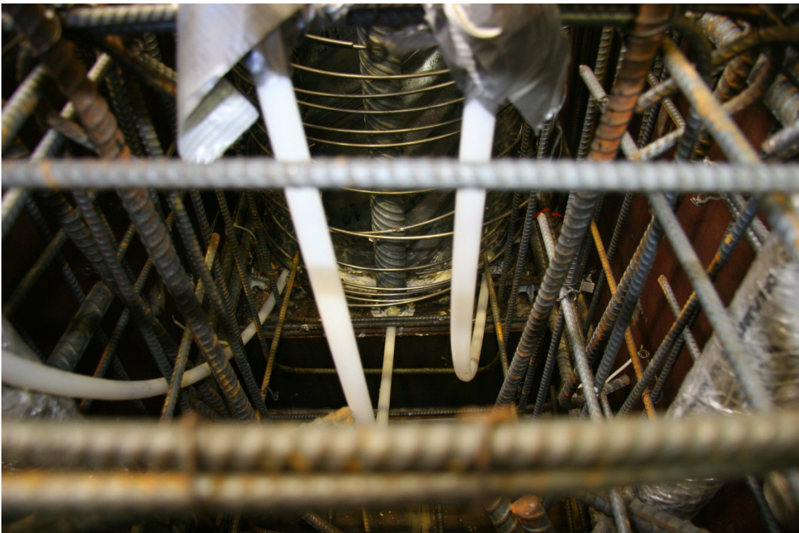
Figure 2.28 Grout tubes running to connection ductwork.
