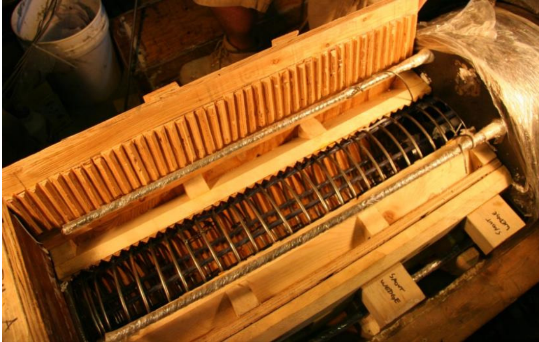
Figure D.4 Formwork for reduced diameter segment.
