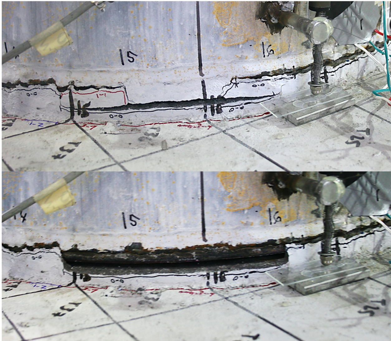
Figure 4.9 Early cracking (top) and removal (bottom) of the cusp underneath the tube weld.
