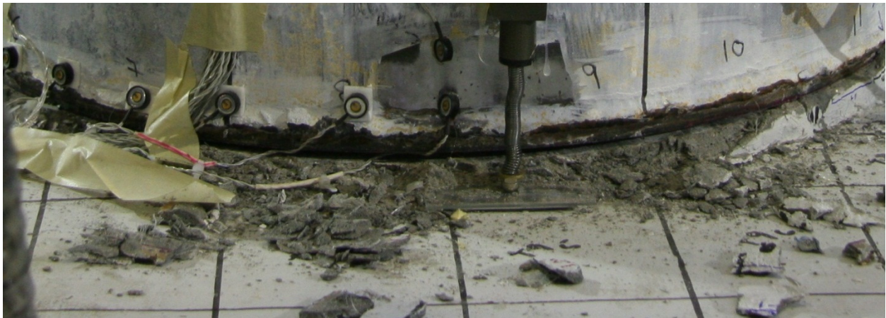
Figure 4.11 Crushing of south side of grout pad resulting from first \pm 10.33\% drift cycle (Set 10-Cycle 2).
