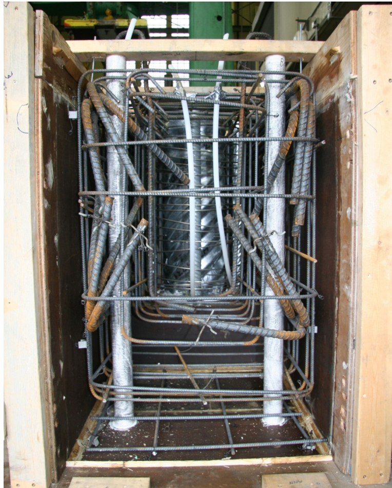
Figure 2.22 End elevation of cap beam reinforcing cage.
