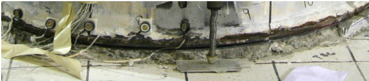
Figure 4.13 South side of grout pad after test completion; note the gap between the baseplate and grout pad caused by permanent compression of the grout.
