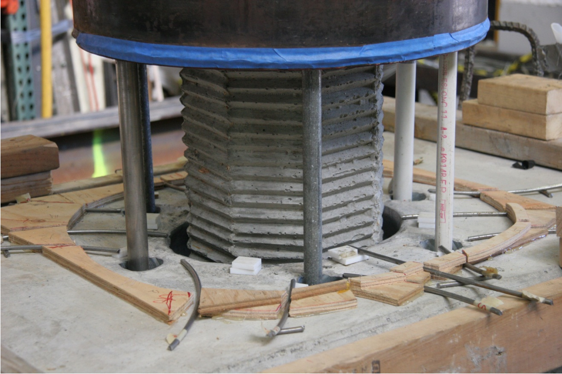
Figure 2.24 Alignment of column extensions into cap beam ducts.
