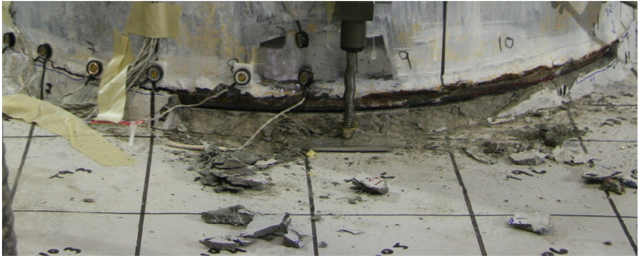
Figure 4.10 Crushing of south side of grout pad resulting from +7.02% / -7.05% drift cycles.
