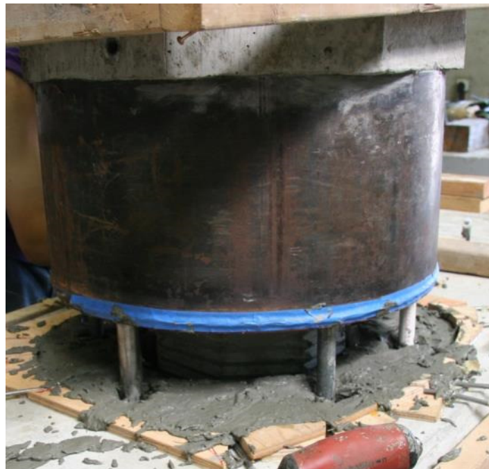
Figure D.14 Placement of fiber-reinforced, 1/2 in. thick, grout pad.
