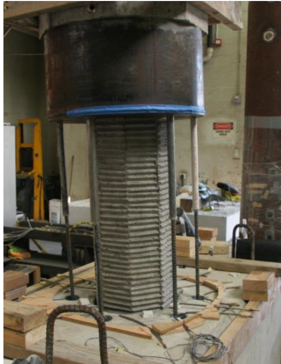
Figure D.13 Fitting of column extensions into cap beam ducts.
