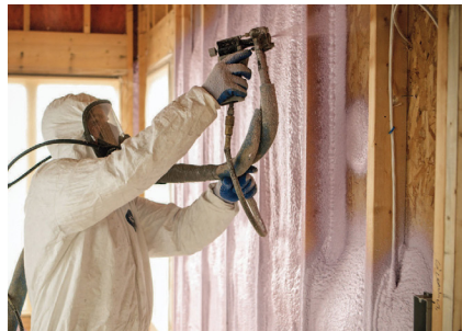
Wood stud wall + spray foam
