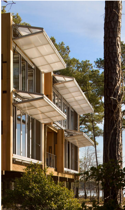
Figure 32: Exterior, Loblolly House Source: https://kierantimberlake.com/pages/view/20/loblolly-house/parent:3
