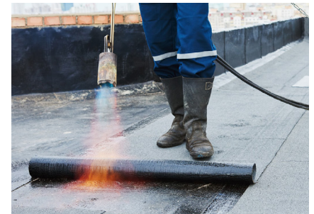
Torch down roofing
