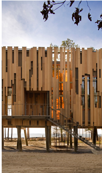
Figure 33: Exterior, Loblolly House Source: https://kierantimberlake.com/pages/view/20/loblolly-house/parent:3
