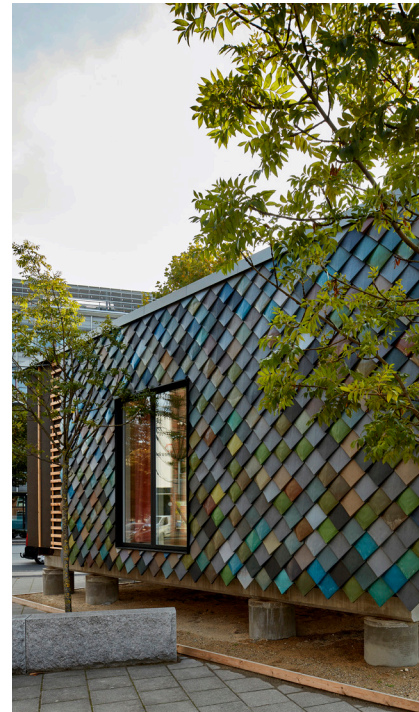
Figure 26: Circle House Facade Construction
