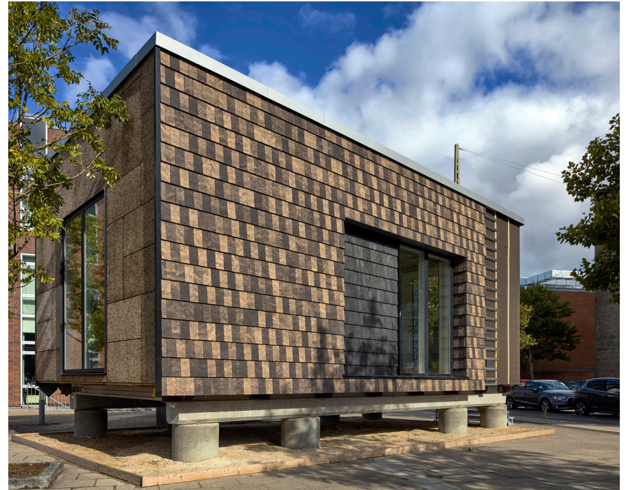
Figure 21: Exterior, Circle House Demonstrator
