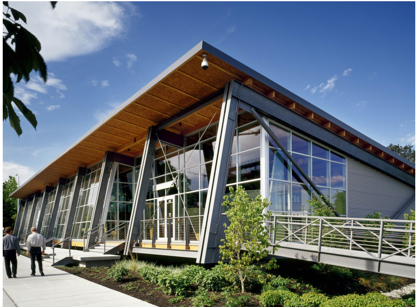
Figure 15: SLU Discovery Center Source: https://www.mutualmaterials.com/projects/south-lake-union-discovery-center/
