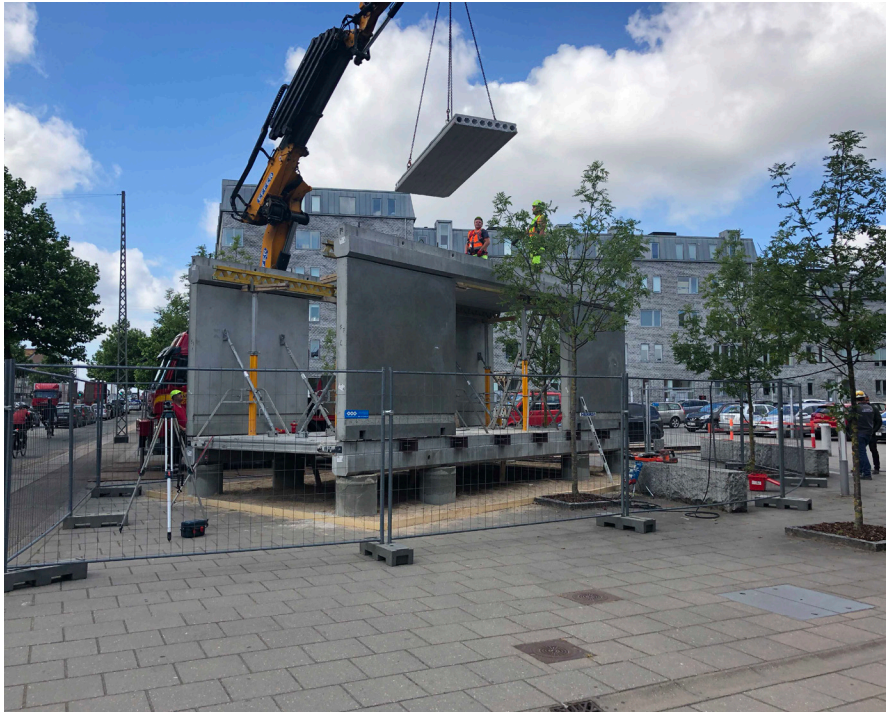
Figure 25: Circle House Demonstrator under construction
