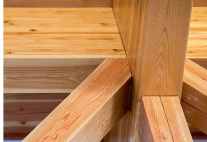
Heavy timber structure
