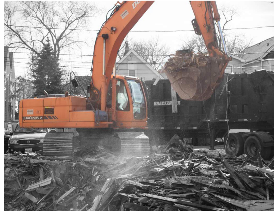
Figure 1: Destructive Demolition http://interactive.wbez.org/curiouscity/chicago-teardowns/
