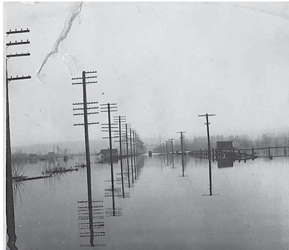
Figure 2.4 Flooded streets in Renton, 1926
